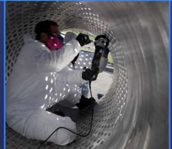
Sleeve Valve Refurbishment
