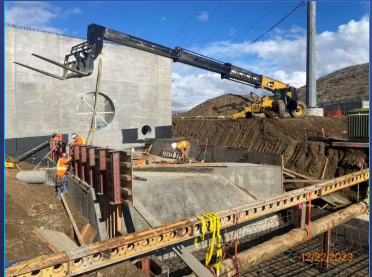
Wadsworth Bypass Pipeline
