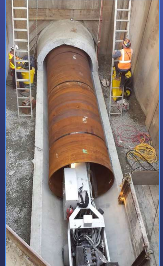
Second Lower Feeder Rehab
