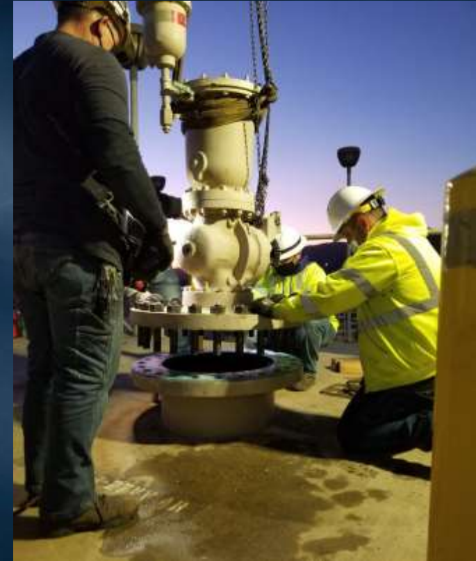
Installing an Air Release/Vacuum Valve at Live Oak Reservoir
