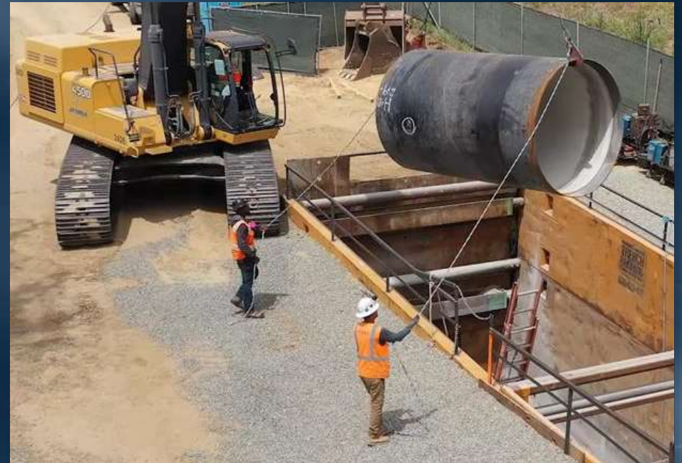
Allen-McColloch Pipeline PCCP Relining
