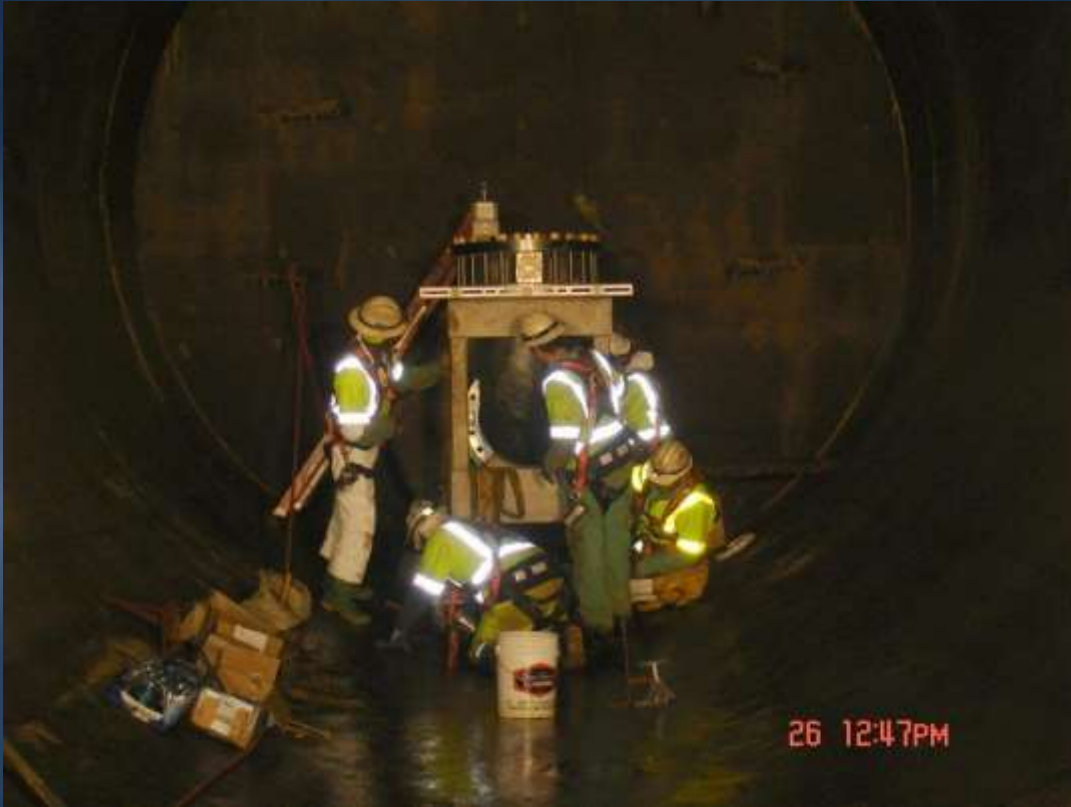
Installing Butterfly Valve in the Foothill Feeder
