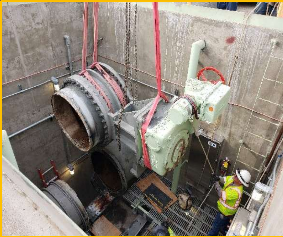
MWD staff remove old 42-inch butterfly valve
