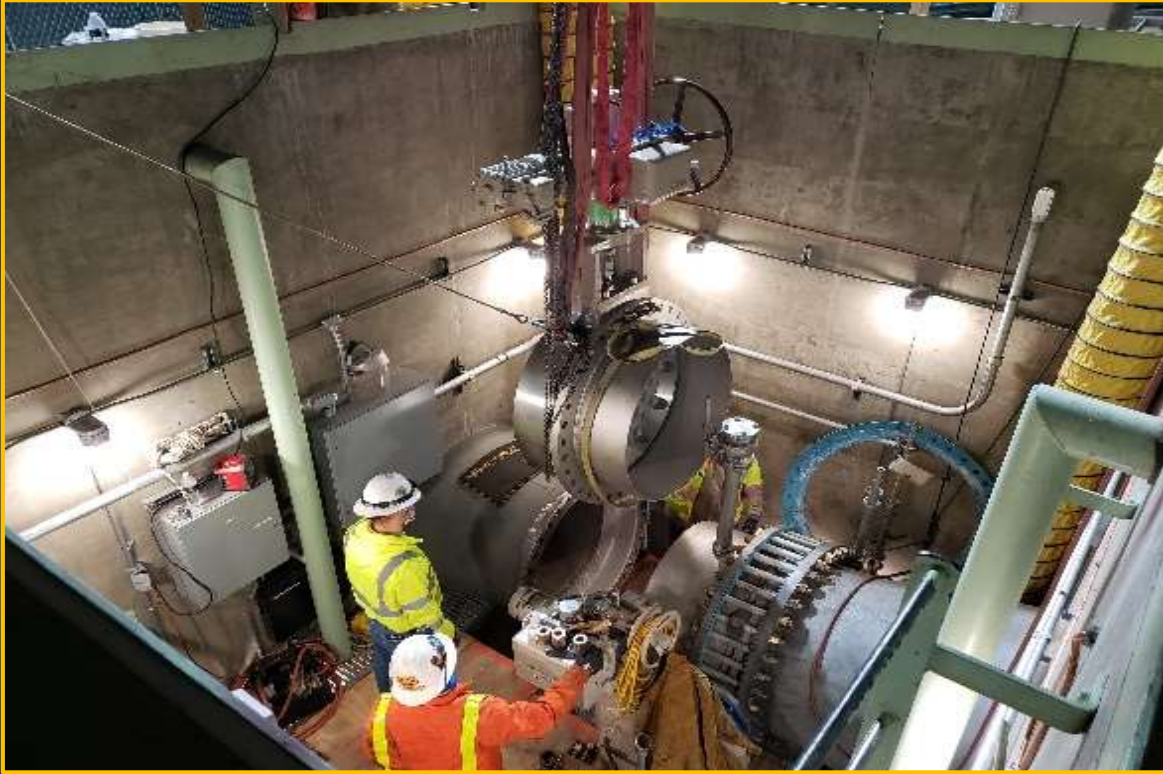
MWD staff install new 42-inch multi-orifice valve
