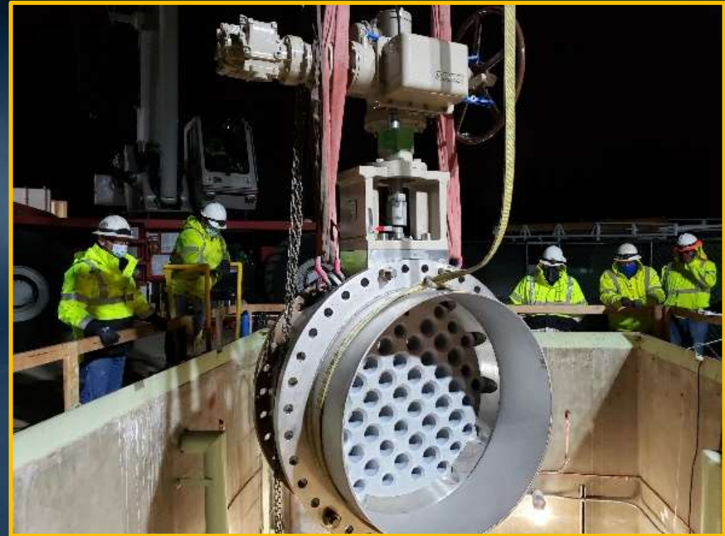
Installation of new 42-inch multi-orifice valve
