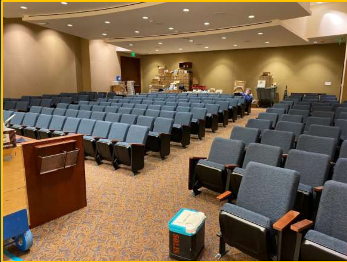
Board Room refurbishments
