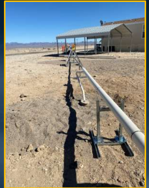
Temporary pump and piping
