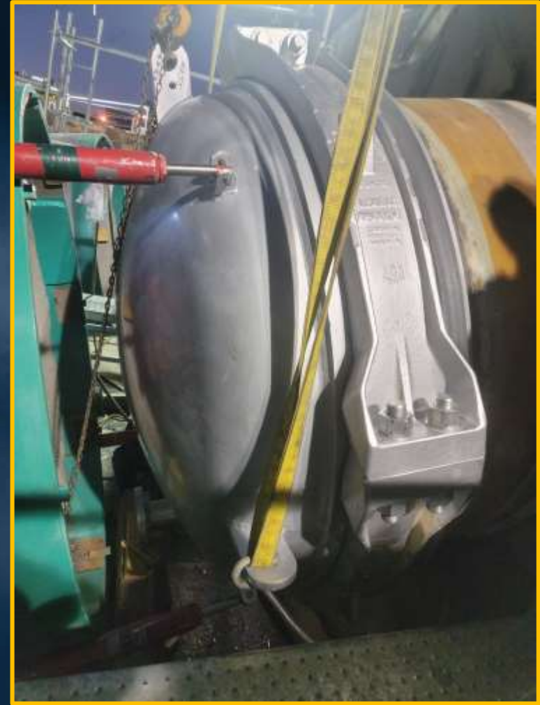
Test fitting of new Isolation Bulkhead
