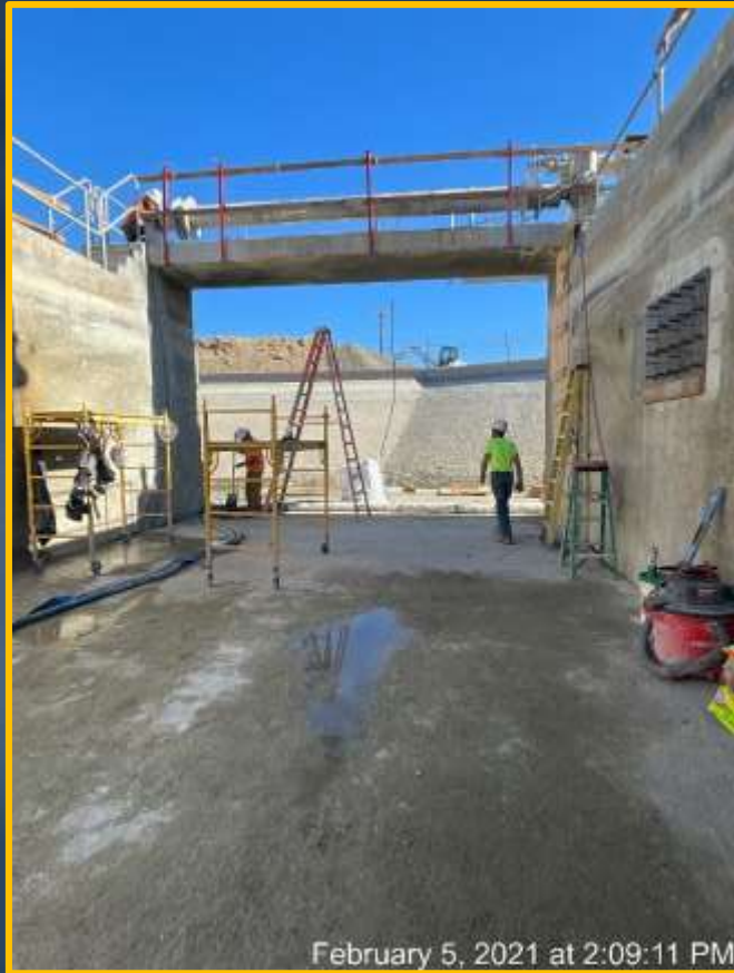
Preparing channel for gate installation
