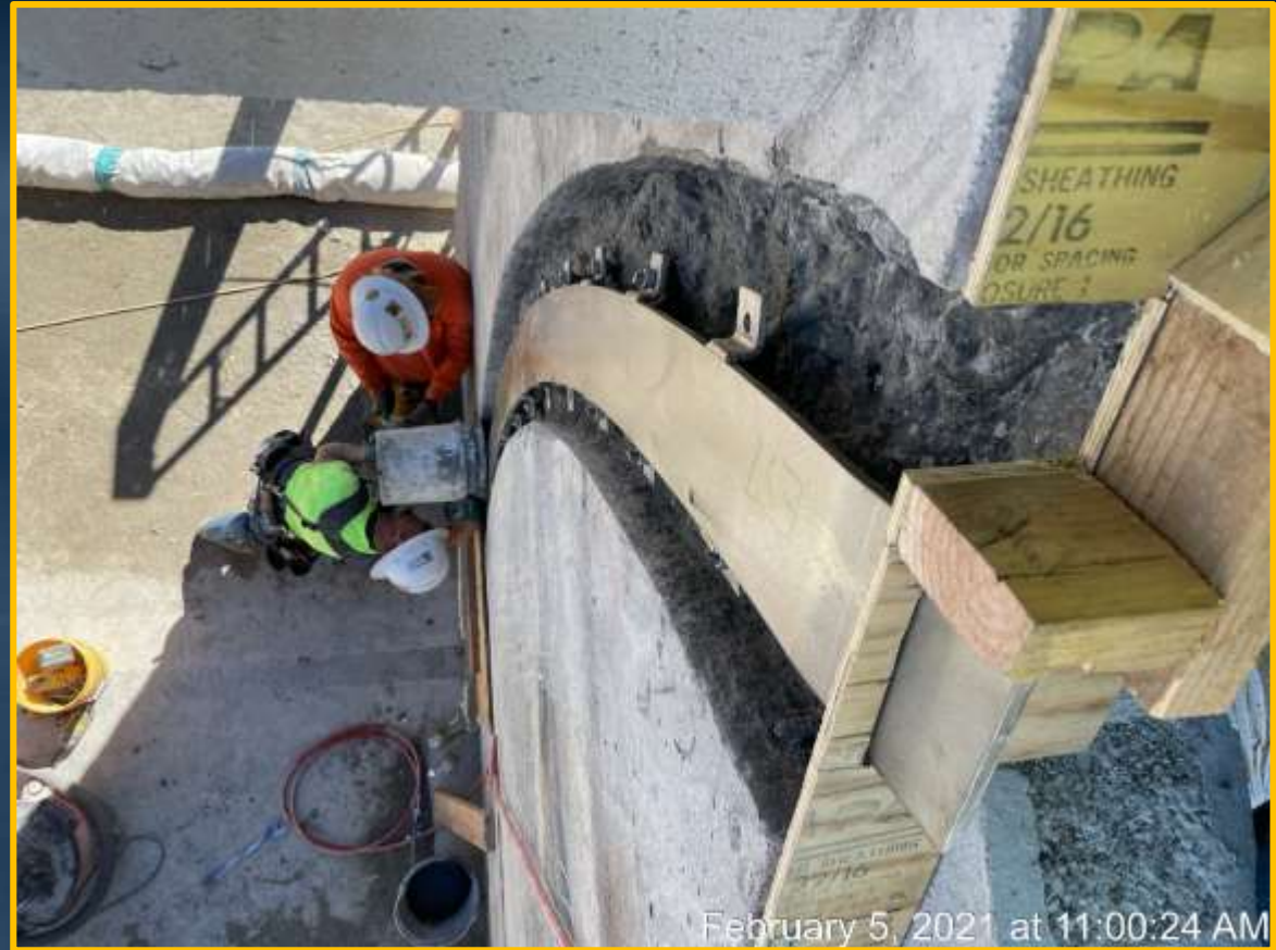
Installation of new gate guide plates
