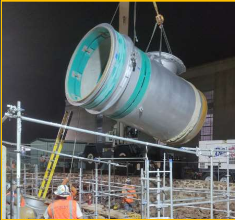
Installation of new Discharge Coupling
