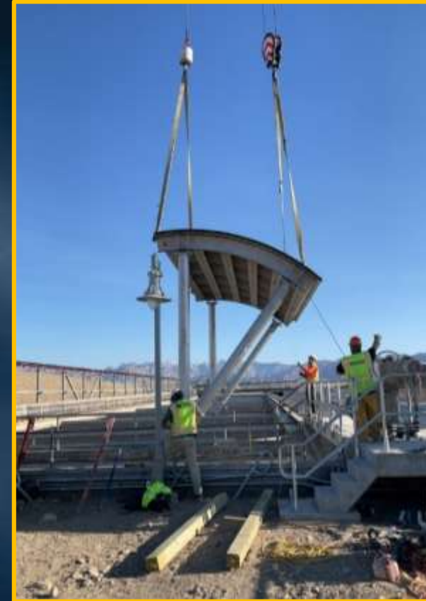
Radial Gate Installation
