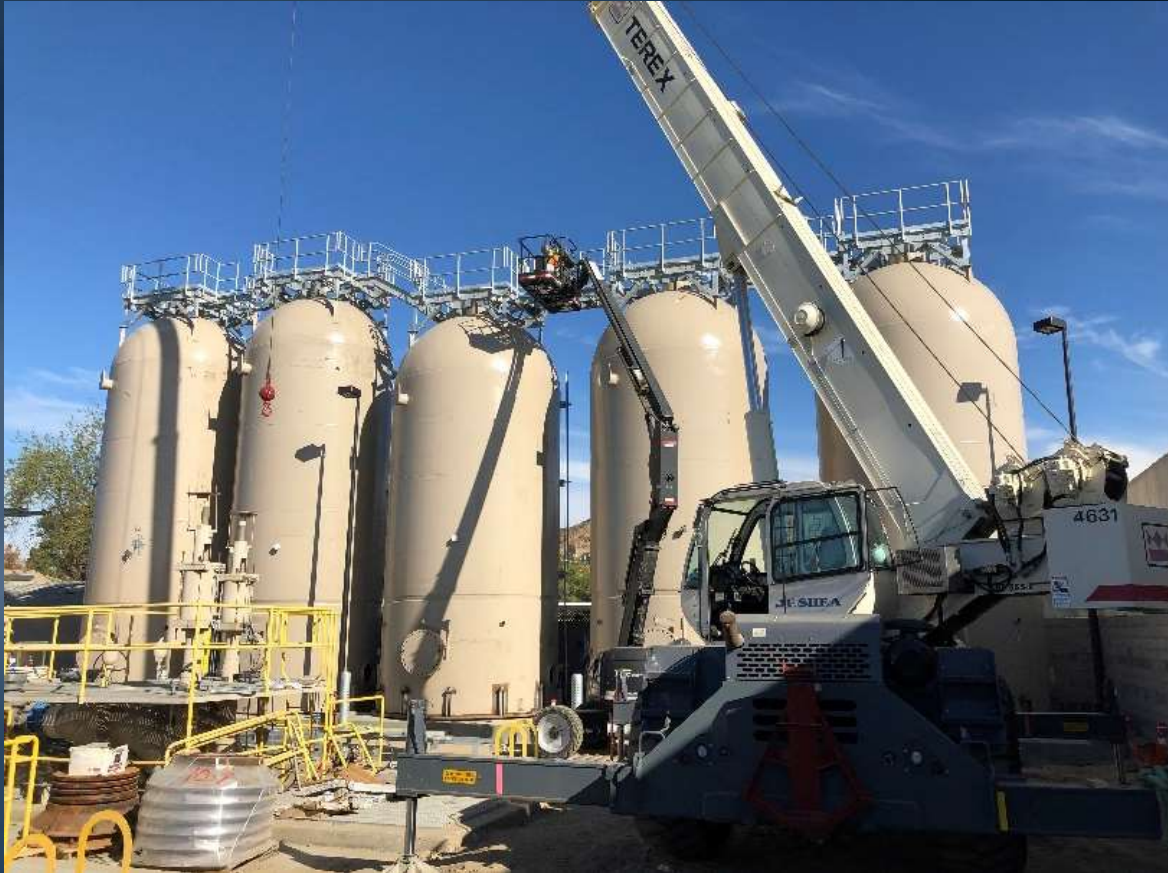
Installation of Surge Tank Catwalk
