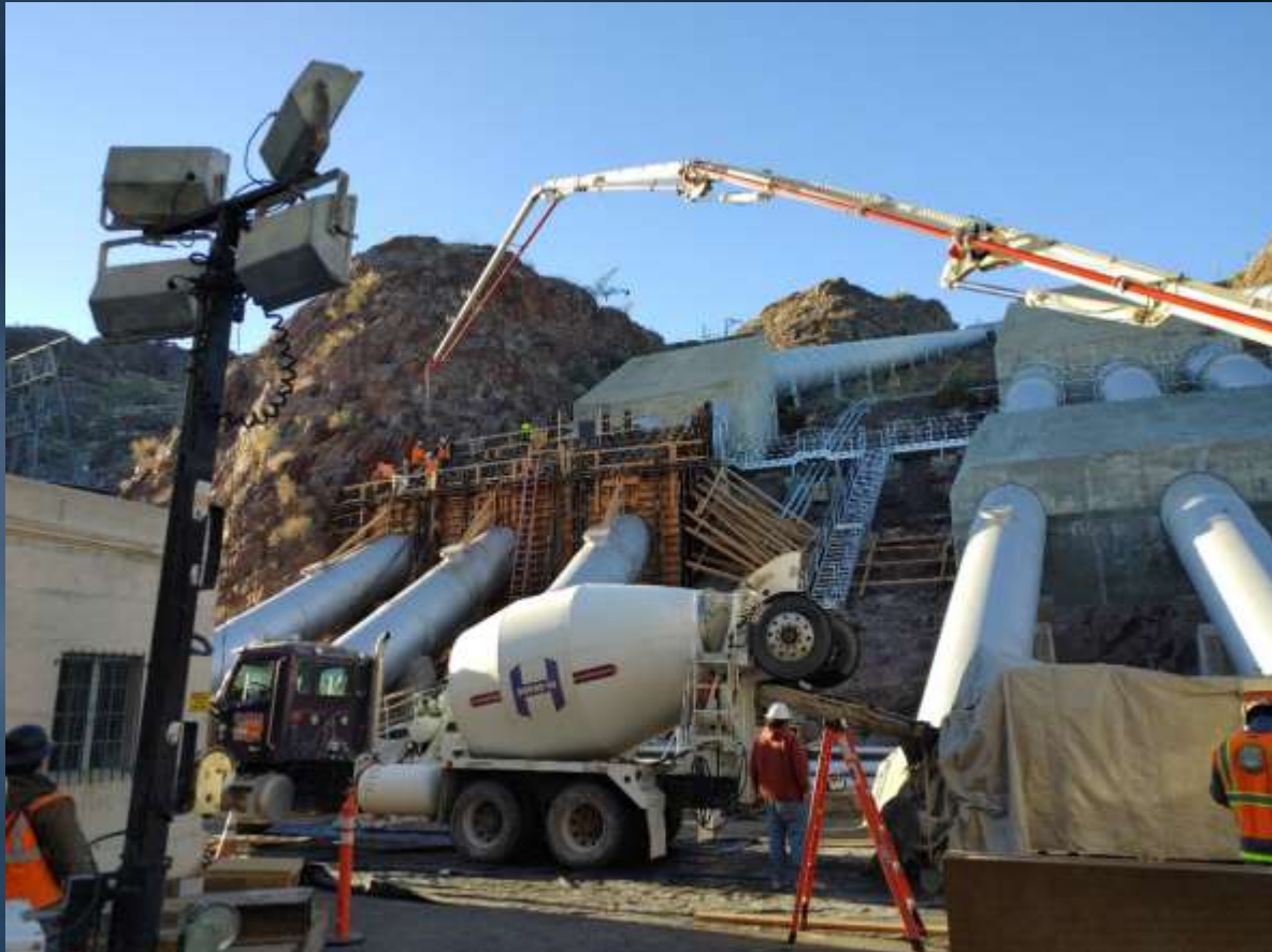
Concrete Placement of New Anchor Block at Intake Pumping Plant
