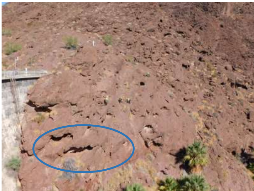
CRA Gene Wash and Copper Basin Discharge Valve Rehabilitation—Rock scaling at Gene Wash Dam
