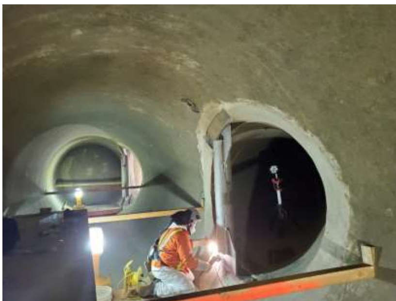
Staff welding prefabricated reinforcements into place at the Perris Pumpback facility
