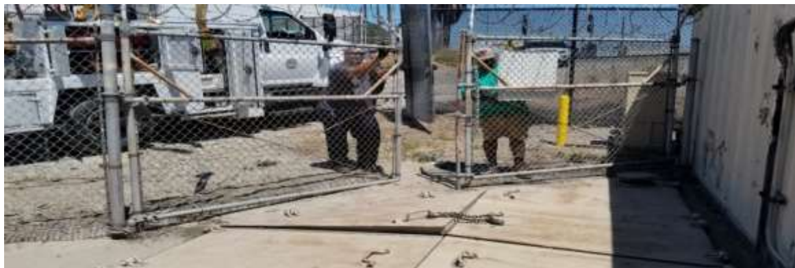
Washington Pressure Control Structure physical security upgrades
