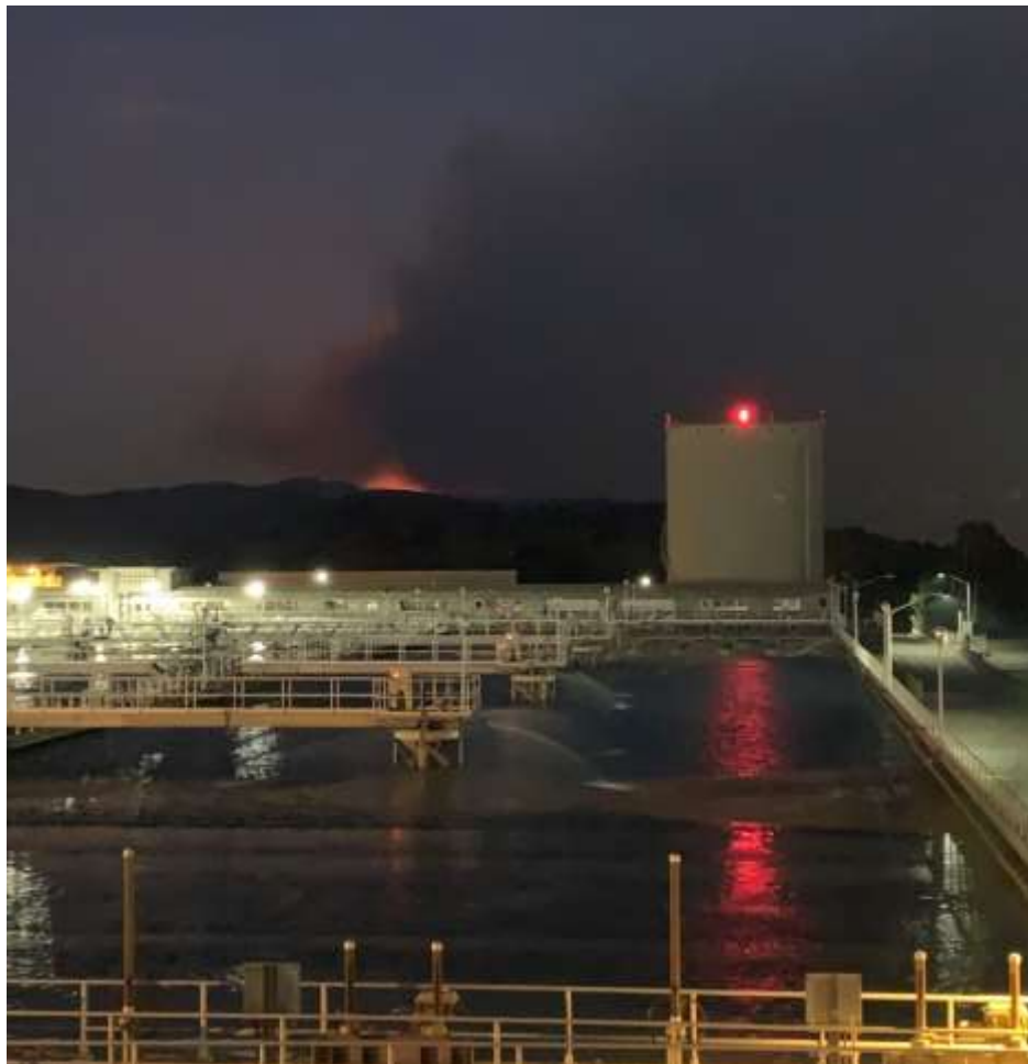
View of the Blue Ridge Fire from the Diemer plant
