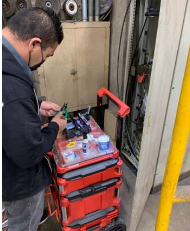
Fiber Splicing - Field Location
