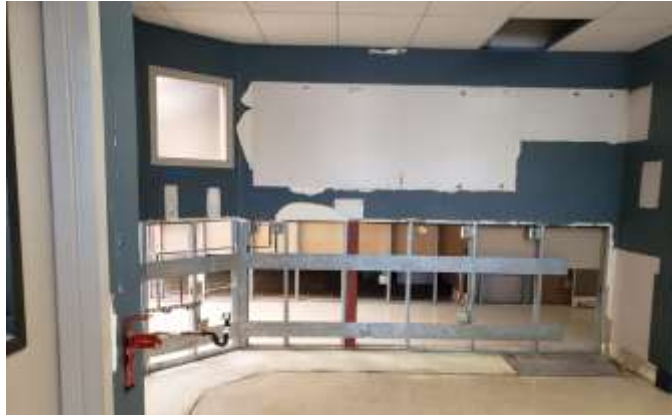
Mills plant breakroom during remediation work
