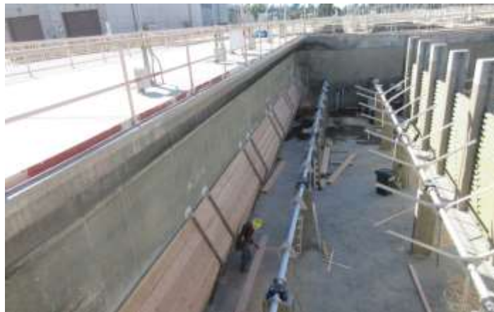
Jensen Module 2 and 3 Flocculator Rehabilitation—Installing inlet baffle board in Basin 5
