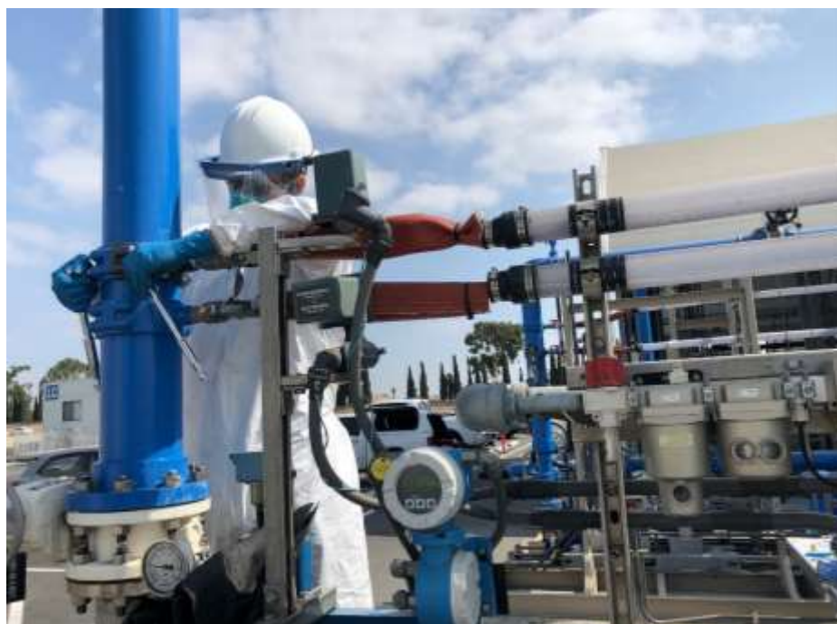
Staff repairing a leaking chemical injection fitting at the demonstration facility
