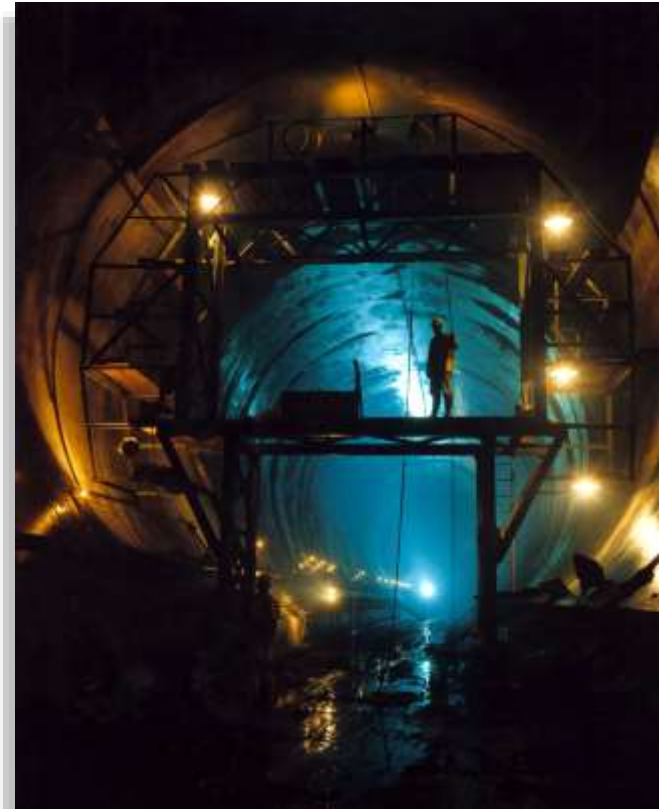
CRA Tunnel Construction
