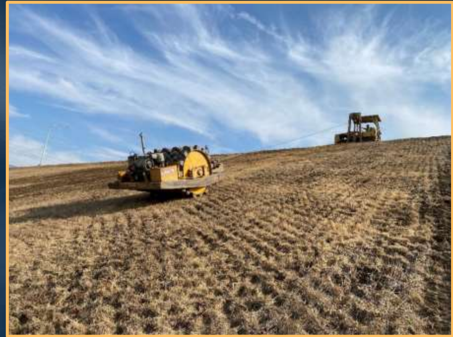
Topsoil Replacement – Compaction Rolling
