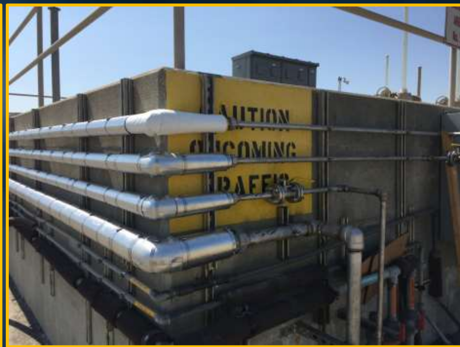
New Stainless Steel Piping
