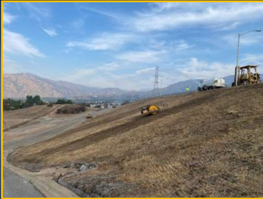
Topsoil Replacement – Compaction Rolling
