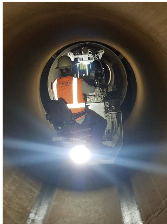
Second Lower Feeder – Reach 8: Pipemobile transporting pipe
