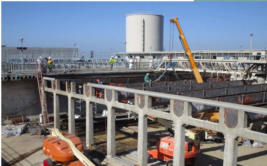
Diemer West Basin No. 7: Removal of existing launders
