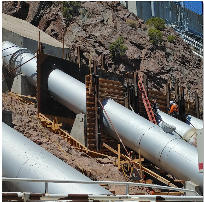
Intake Delivery Line No. 3 concrete anchor block formwork
