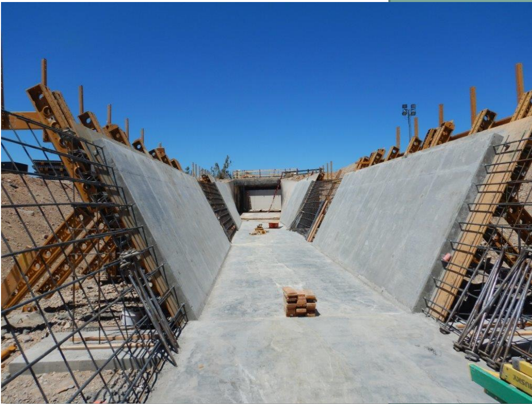
Installation of temporary formwork and reinforced concrete at Vidal Wasteway
