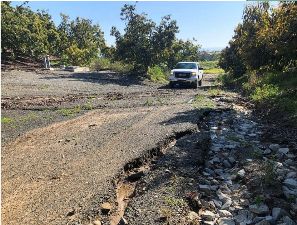
Access road to be improved along Allen-McColloch Pipeline
