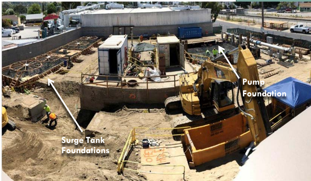
Surge tank and pump foundations
