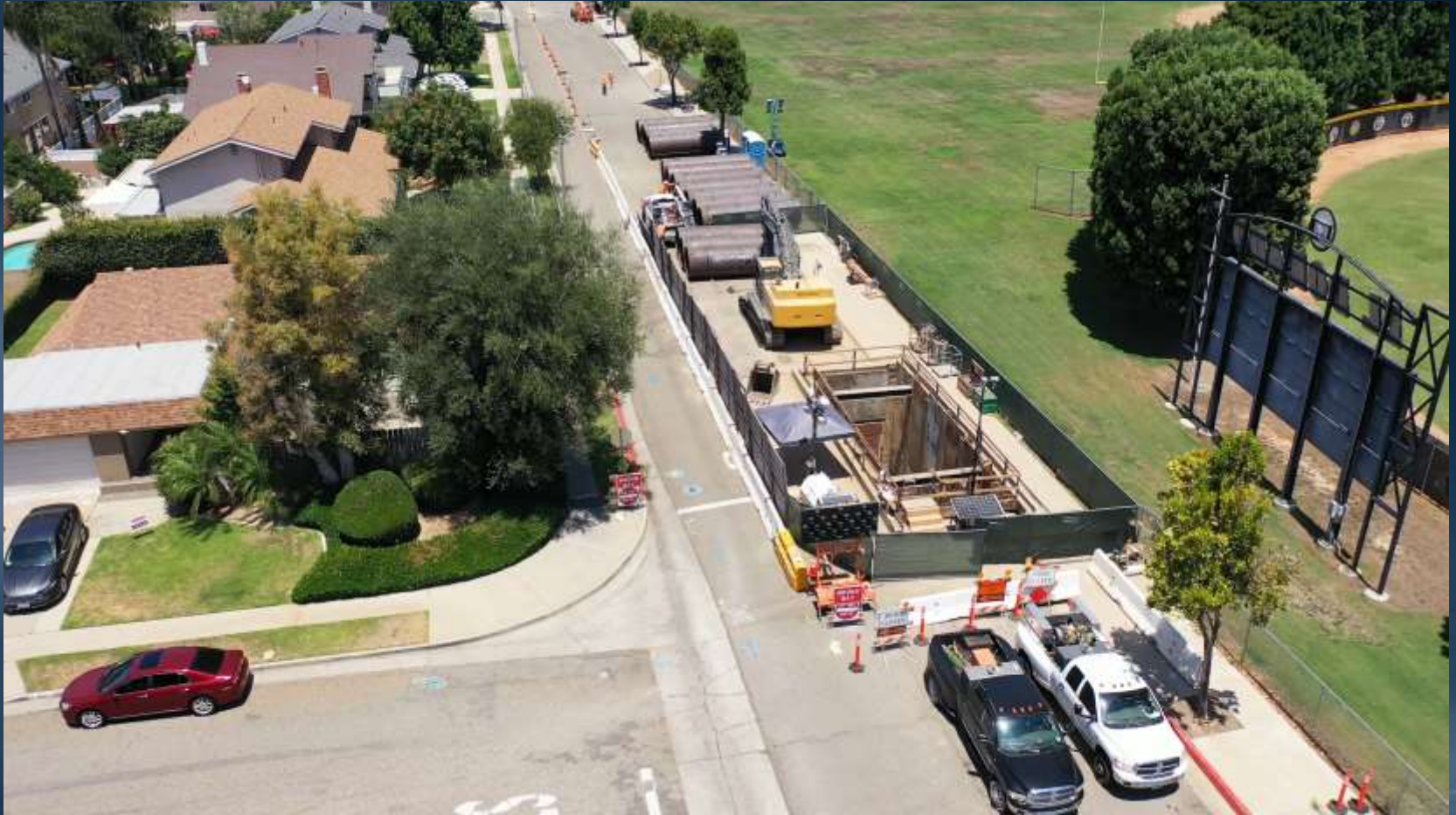
Reach 8 Pipe Placement
