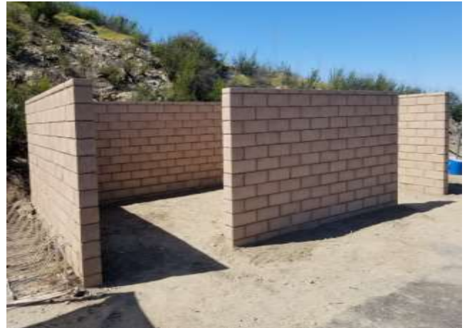
After DVL Viewpoint restroom facility renovation
