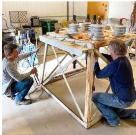
Staff servicing transformer bushing prior to installation at Gene pumping plant
