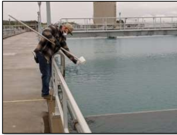
Staff collecting water samples from the sedimentation basin at the Diemer plant
