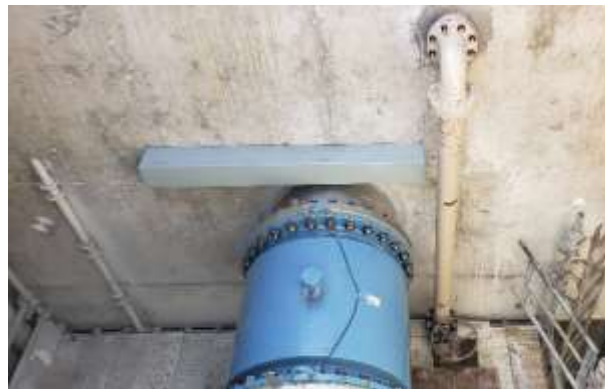
Completed installation of meter for SKPE-1 service connection
