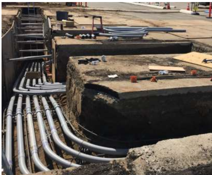
Weymouth Water Quality Instrumentation Improvements – Installation of duct bank conduit
