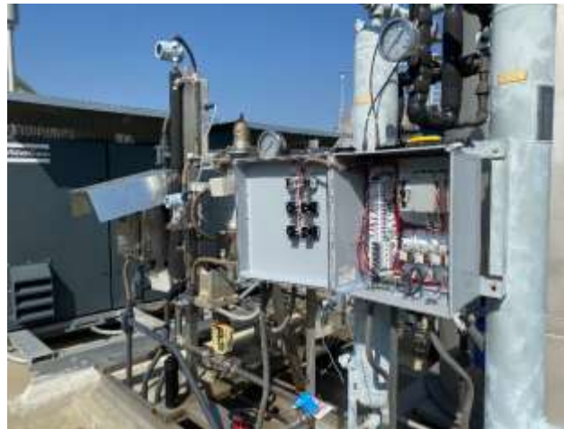
Nitrogen dryer PLC upgrade at the Jensen plant
