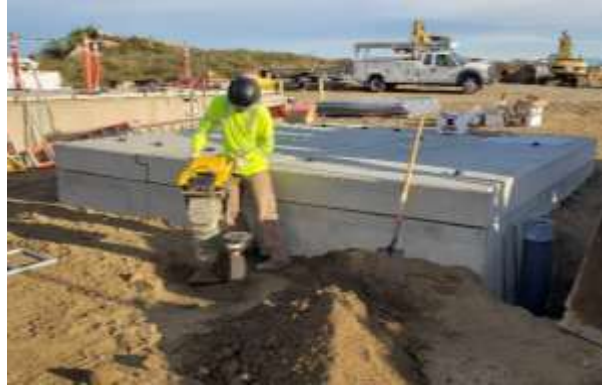
Staffing backfilling upstream vault air release valve for SKPE-1 service connection
