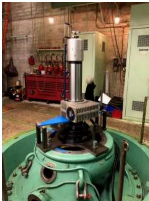
Setup to machine a pump seal ring at Gene pumping plant
