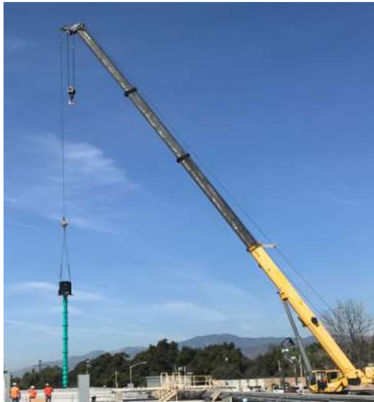
Weymouth Domestic Water Upgrade – Setting of Domestic Water Pump No. 2
