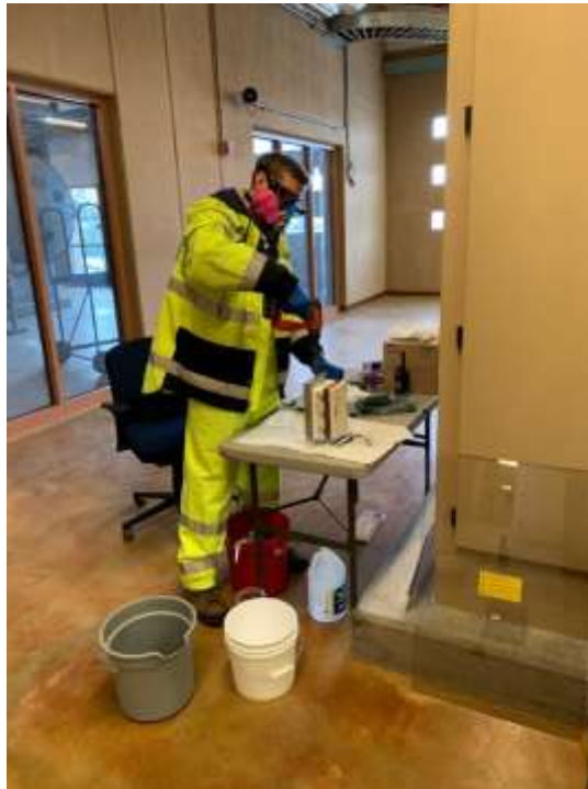
Staff refurbishing an ozone PSU transistor at the Skinner plant
