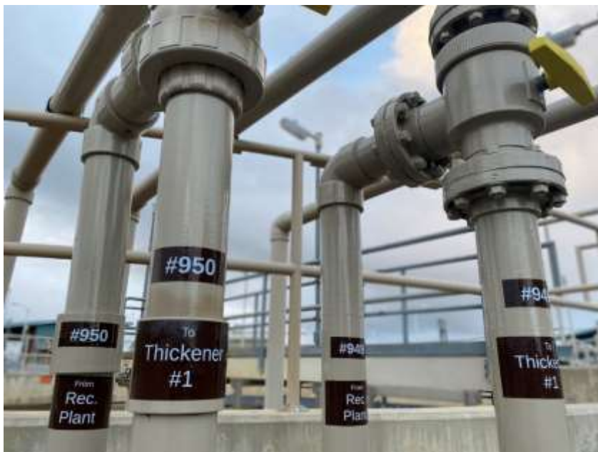
Re-coated and re-labeled thickener manifold piping at the Skinner plant
