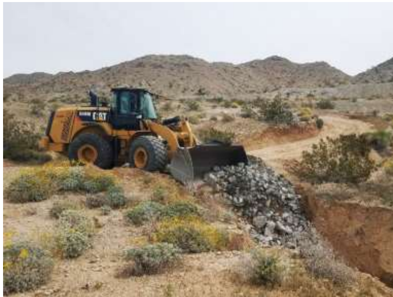
Staff repairing a CRA patrol road damaged by storms
