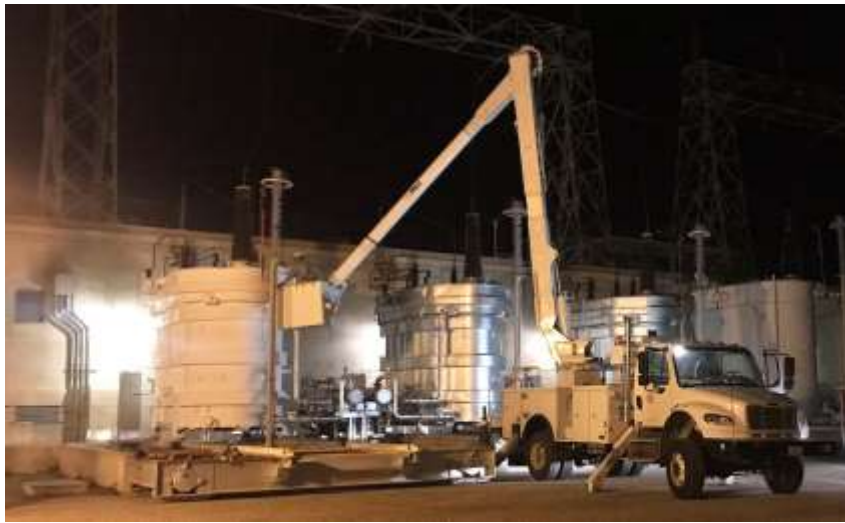
Staff bringing a spare transformer into service at Gene pumping plant
