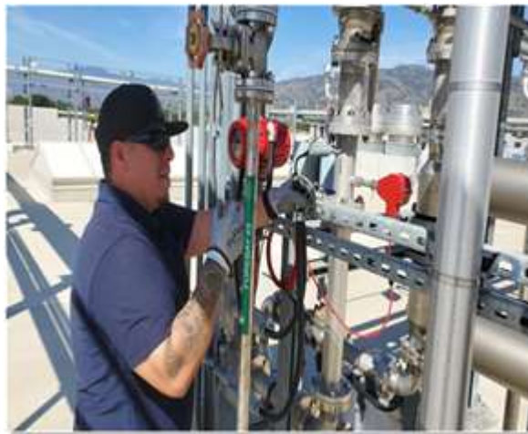
Staff installing new flow meter at the Weymouth plant.
