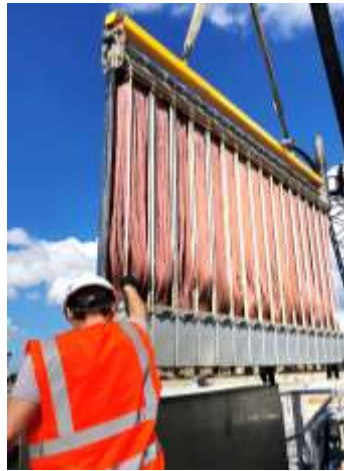
Installation of membranes for the MBR system following maintenance repairs
