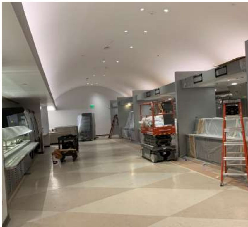
Headquarters Building Improvements – Remodeled server area with new layout and equipment
