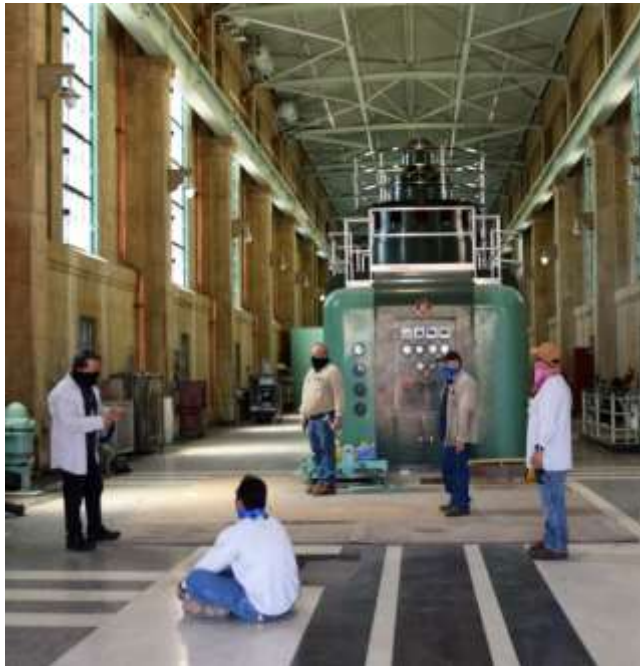
Pre-job toolbox meeting at Hinds pumping plant along the CRA
