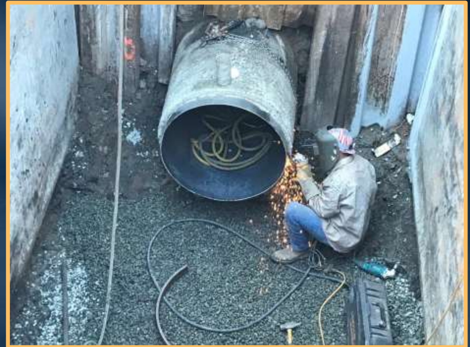
Site 13 – Closure Piece Installation
