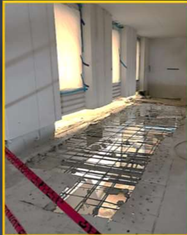
Level 5 Roof Deck Demo
