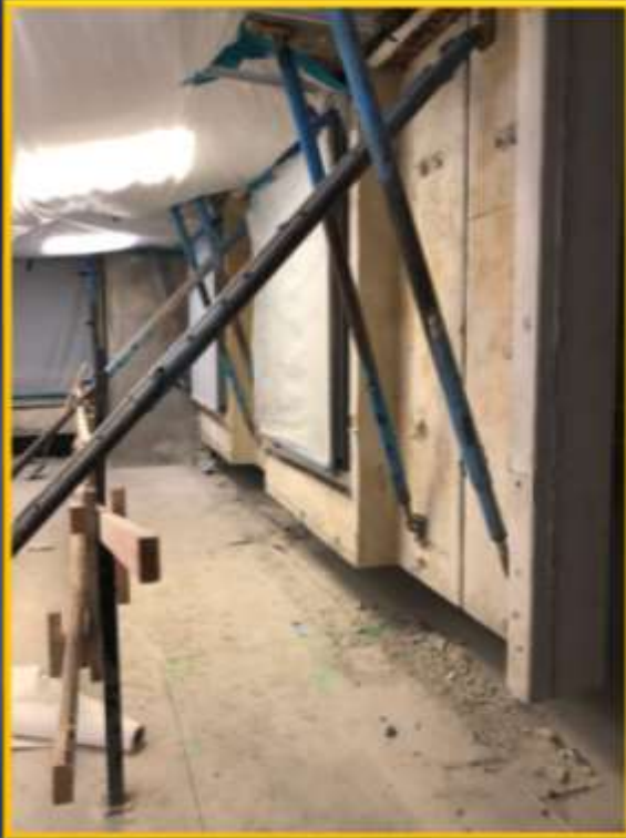
Cladding Panel Bracing for Level 6 Tower
