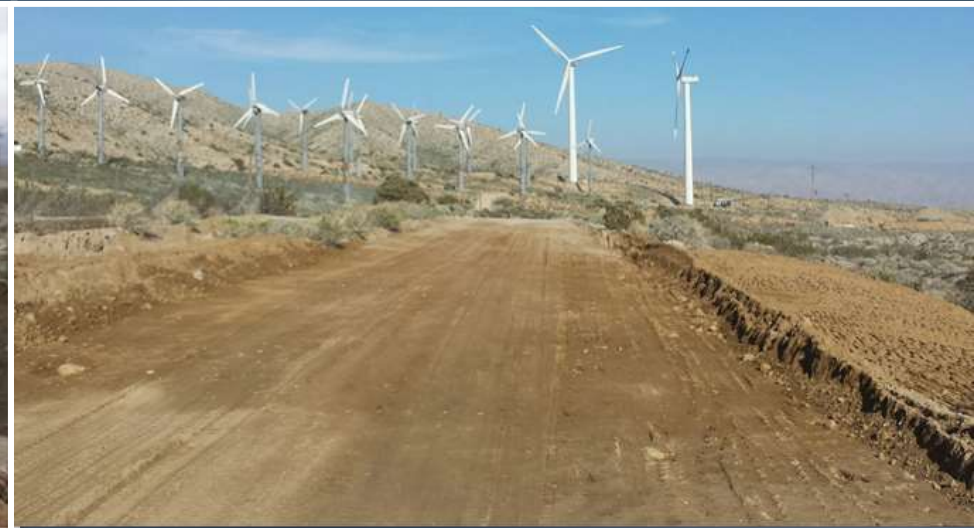
Repaired Patrol Road
