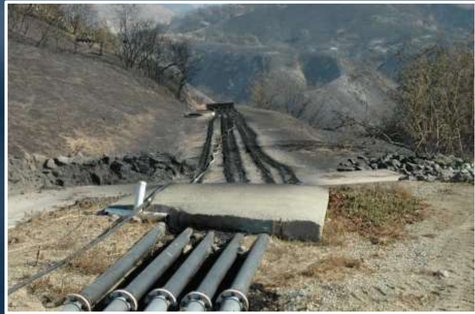
Fiber Optic Cable at Diemer - 2008
