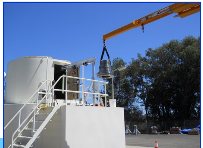
Staff removing equipment for refurbishment at Red Mountain Hydroelectric Plant
