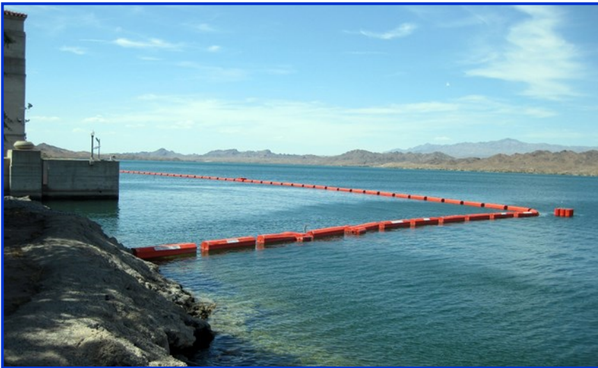
New demarcation floating barrier at Whitsett Intake pumping plant on Lake Havasu
