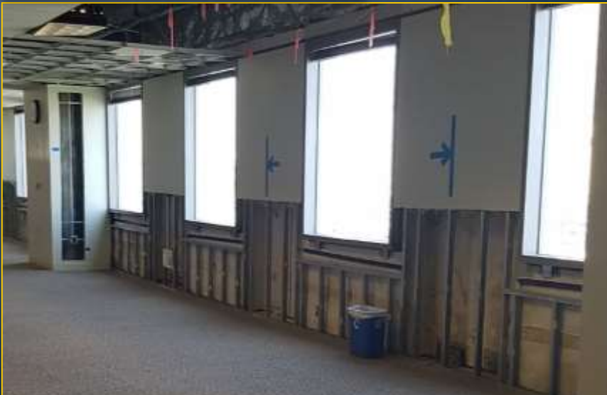
Demolition of Finishes at Wing & Tower
