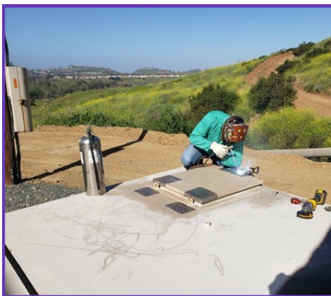
Staff making security improvements at a pipeline structure
