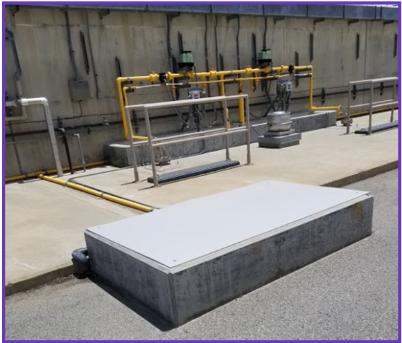
Installed chemical sump cover at the Skinner plant
