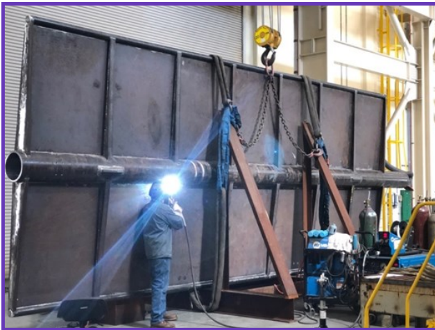
Staff making security improvements at a pipeline structure
