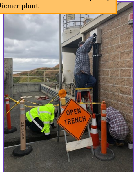
Staff saw cutting asphalt and excavating trench to install water quality sample lines and electrical conduit at the Diemer plant
