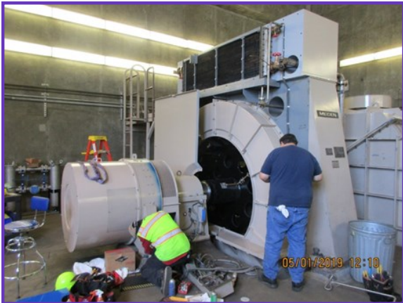
Staff performing final reassembly on the generator at Valley View HEP
