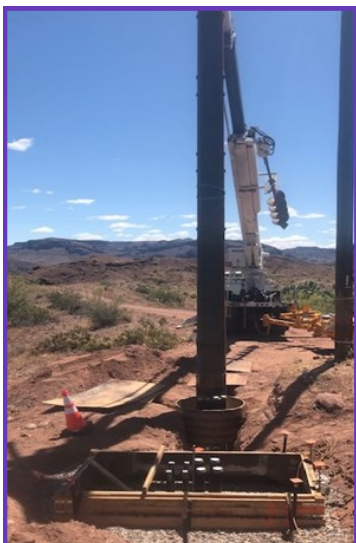
Power pole installation
