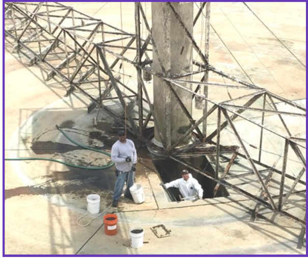
Staff performing maintenance on a sedimentation basin at the Weymouth plant
