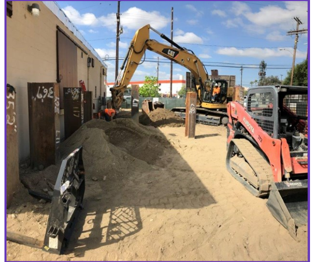
Greg Avenue Pump Station Rehabilitation – Shoring installation near existing control building
