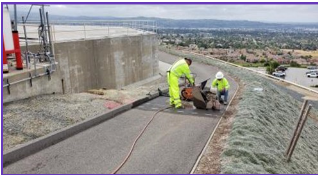
Staff saw cutting asphalt and excavating trench to install water quality sample lines and electrical conduit at the Diemer plant
