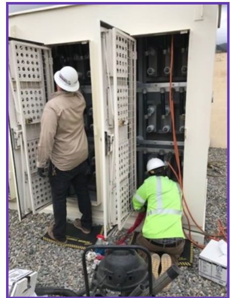
Staff performing maintenance on electrical systems at Corona HEP
