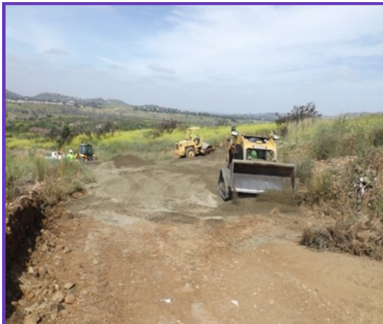
Staff placing aggregate material along Santiago Lateral patrol road
