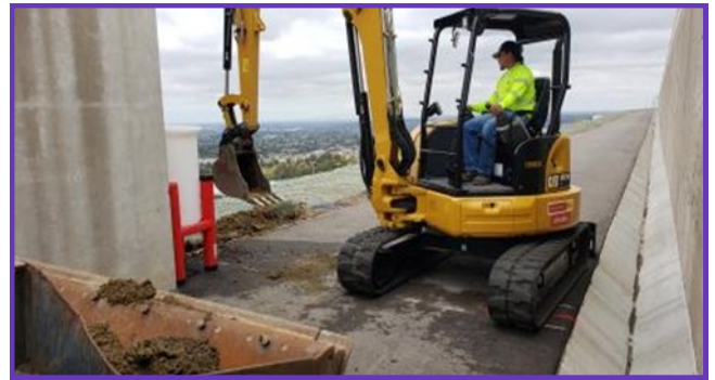
Staff saw cutting asphalt and excavating trench to install water quality sample lines and electrical conduit at the Diemer plant
