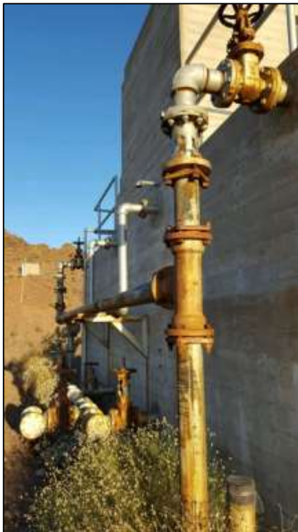
Gene Pumping Plant: Deteriorated asphalt pavement and water piping system
