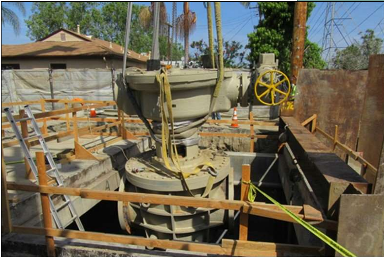
Removal of existing 42" isolation valve for Reach 4
