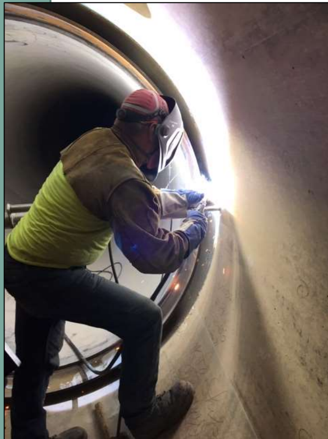
Welding of 20-foot long pipe segment after liner installation
