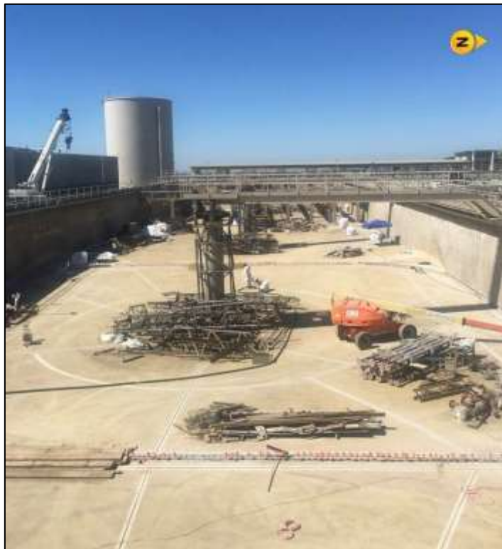
Diemer West Basin No. 5, showing demolition of sludge rakes
