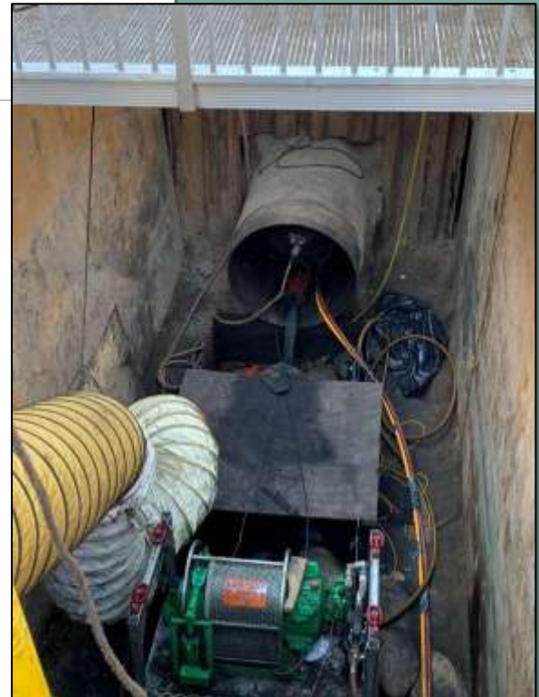
Orange County Feeder: Preparation for removal of coal tar enamel
