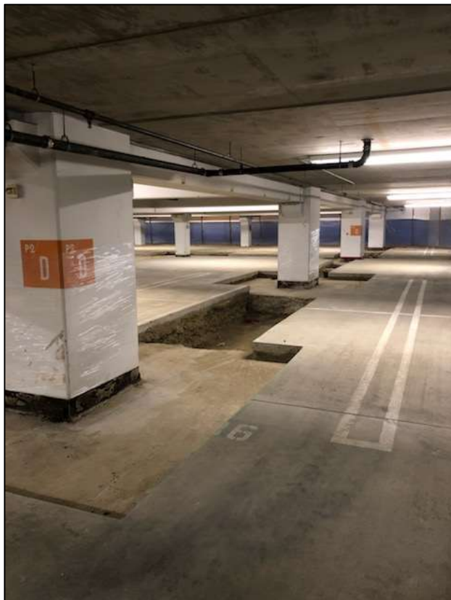
Excavation for grade beams in Union Station parking garage
