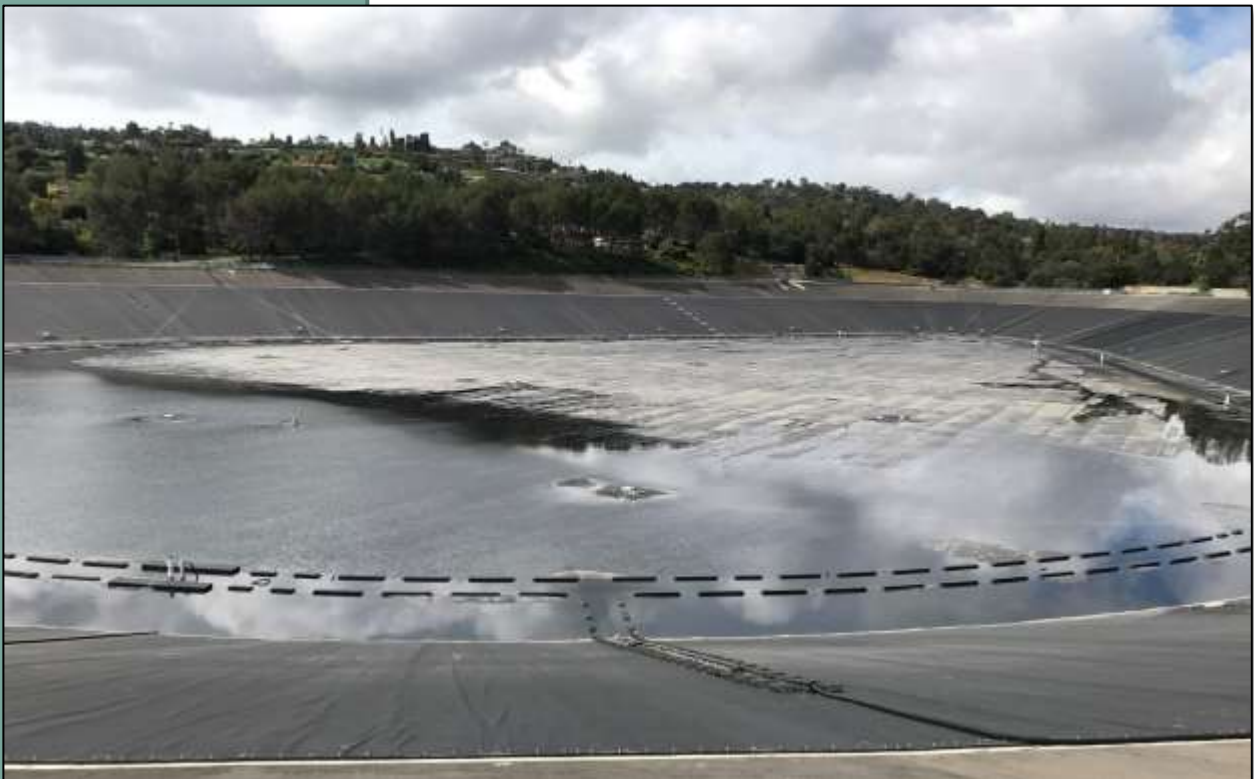
Palos Verdes Reservoir: New floating cover installation complete
