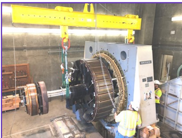
Staff installing the generator rotor at the Valley View Hydroelectric Plant
