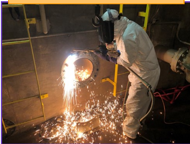
Staff installing new valves at Red Lion Pressure Relief Structure
