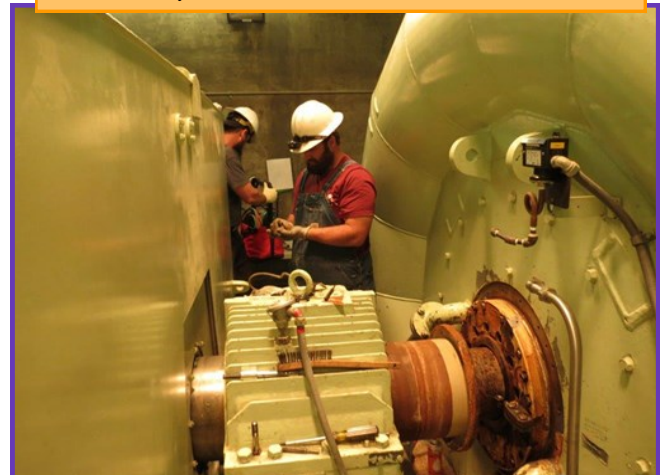
Mechanical apprentice assisting with repairs at the Temescal Hydroelectric Plant
