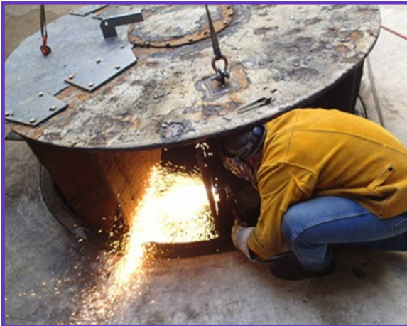
Staff fabricating inlet flow diffuser at Gene pumping plant
