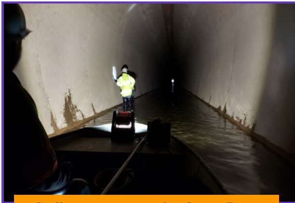
Staff inspecting a tunnel at Copper Basin
