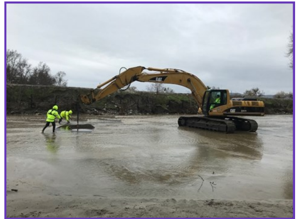
Staff placing k-rail and steel plates to protect pipelines within the San Jacinto River
