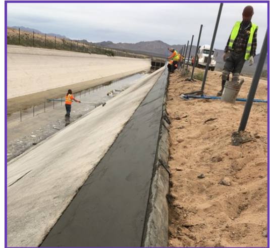
Staff repairing concrete panels along the Colorado River Aqueduct
