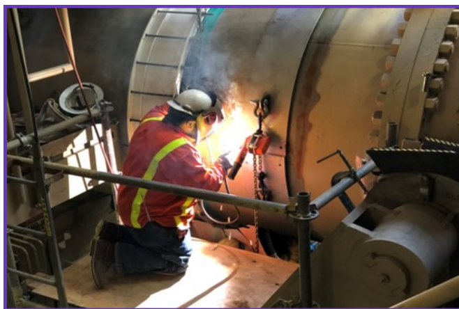
Staff installing a new dresser coupling (l) and pipe section (r) at Red Mountain HEP
