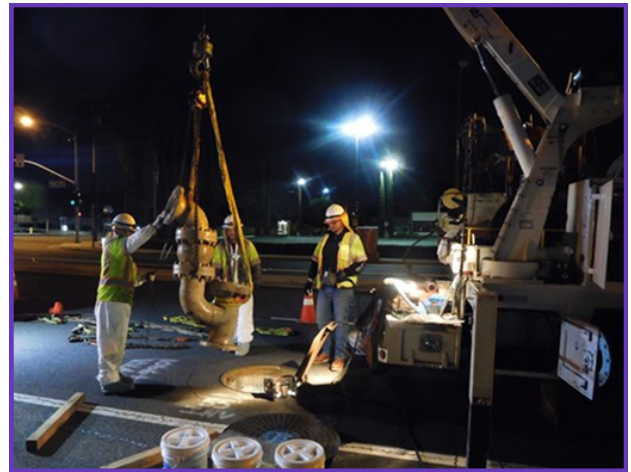
Staff removing equipment to access the Second Lower Feeder]
