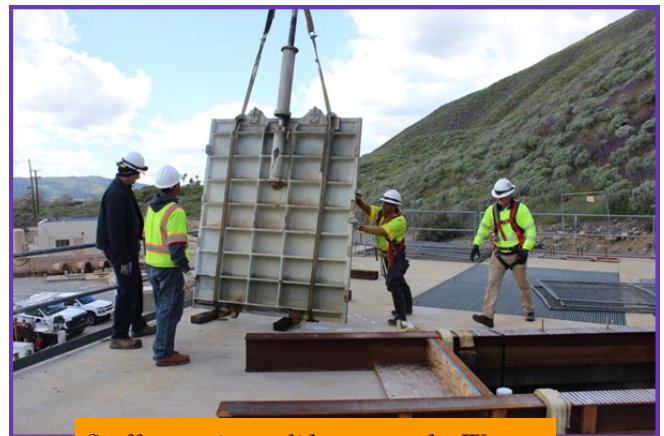
Staff removing a slide gate at the West Portal of the CRA San Jacinto Tunnel
