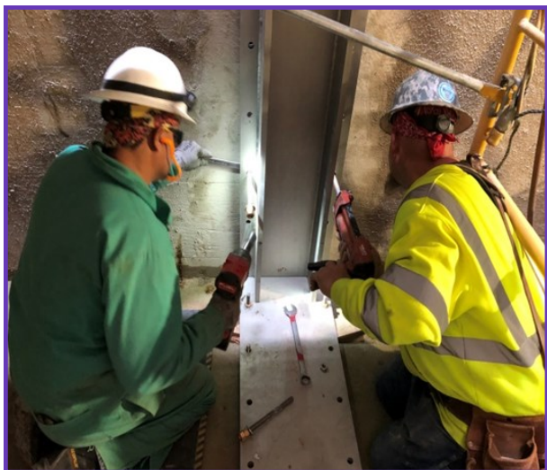
Staff installing new gate guides at the Casa Loma Canal
