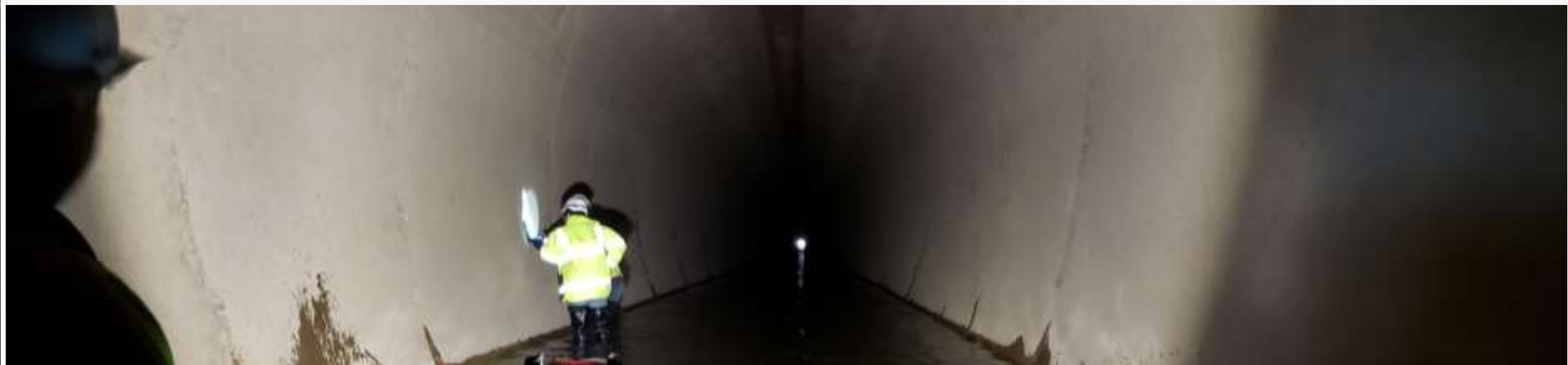
Tunnel, Conduit, Siphon Inspections
