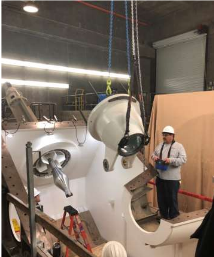
Installing Needle Valve
