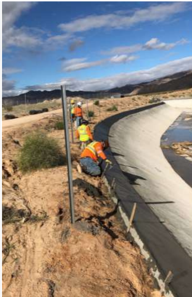
Canal Liner Repairs
