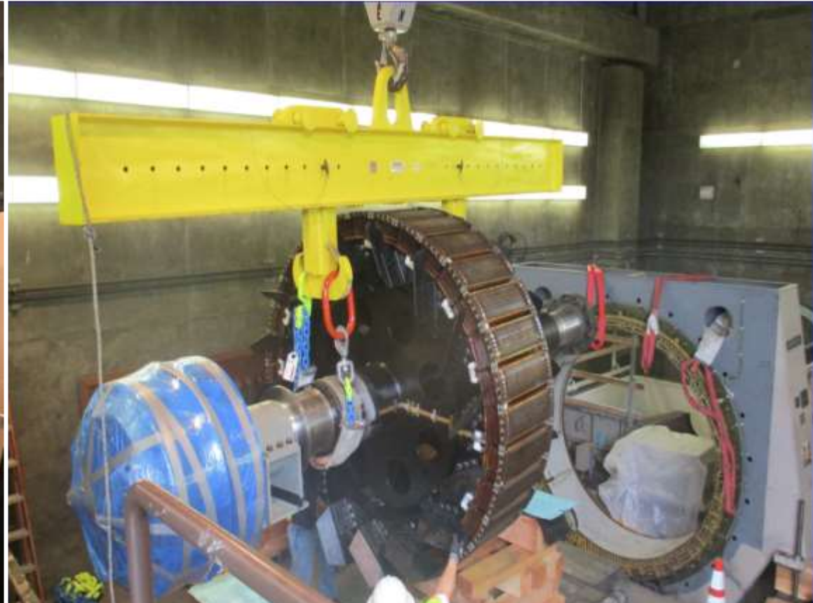
Installing Generator Rotor
