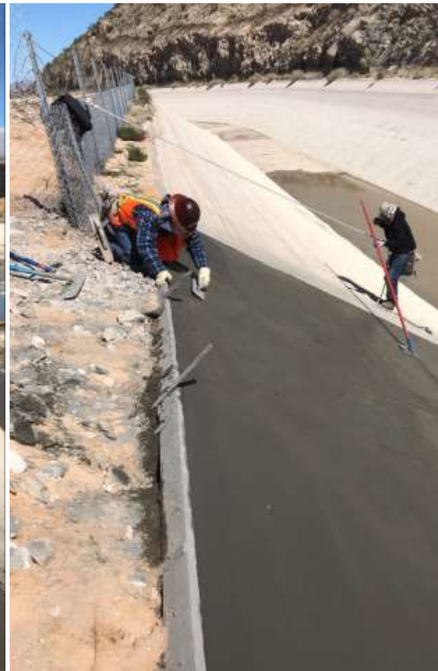
Canal Liner Repairs
