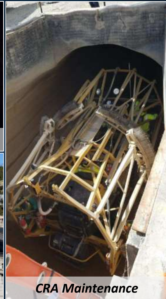
Second Lower Feeder PCCP Relining
