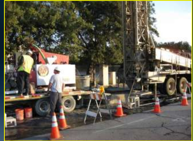
Drilling of anode well
