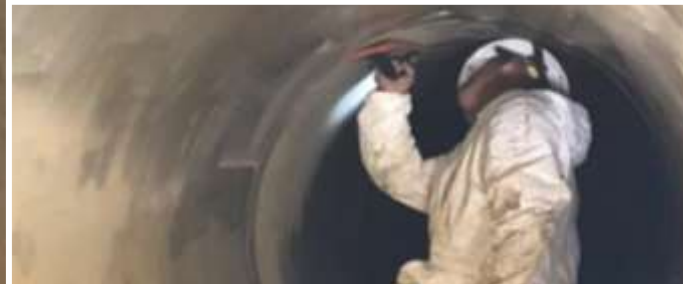
Mortar Lining Repair
