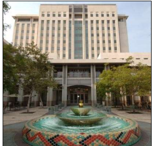
Metropolitan’s Headquarters Building at Union Station
