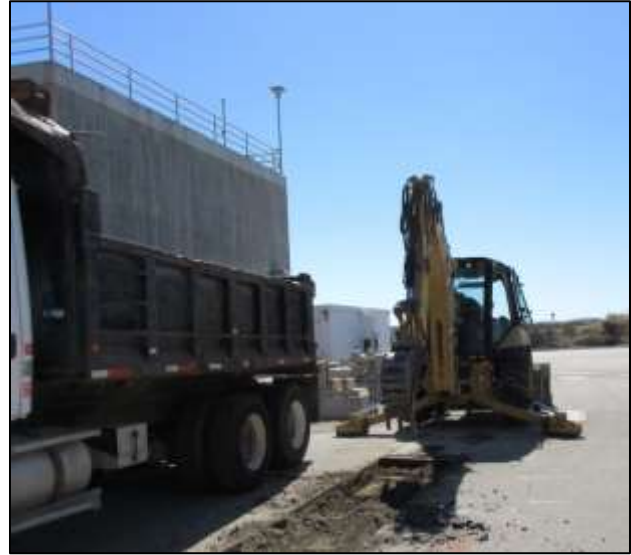
Mills Electrical Upgrades Removal of asphalt for ductbank excavation
