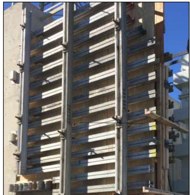
Switch House Building Seismic Upgrades Buttress wall forms
