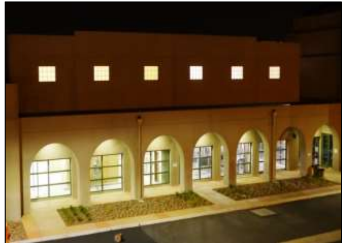
Weymouth Plant Ozone Generation Building
