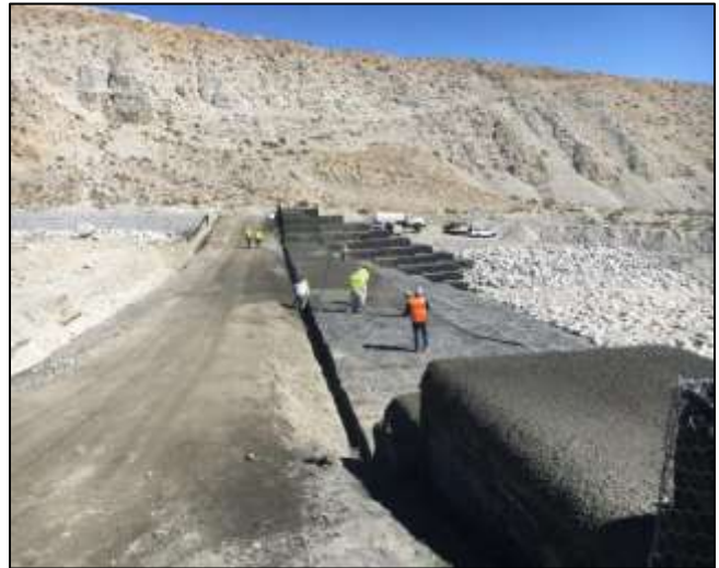
Whitewater Siphons Erosion Protection Spraying of shotcrete on the drop structure
