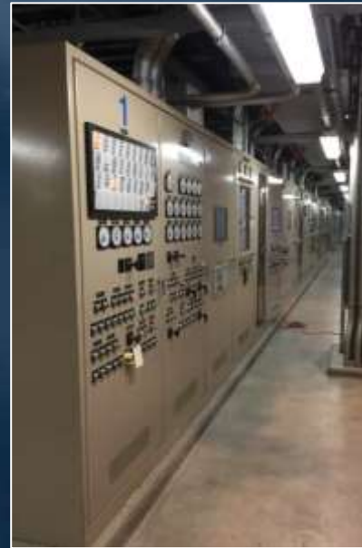
Wadsworth PP Pump and Turbine Control System Equipment
