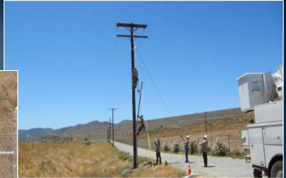
Power line and pole installation
