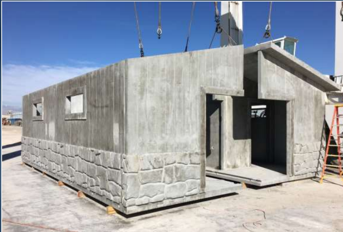
New prefabricated concrete restroom facility
