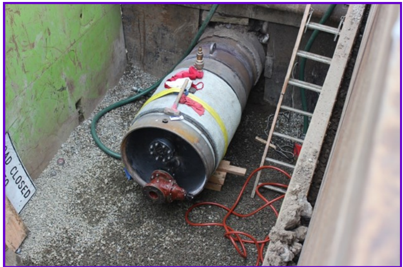
Orange County Feeder before (left) and after (right) the bulkhead installation to keep the majority of the feeder in service.
