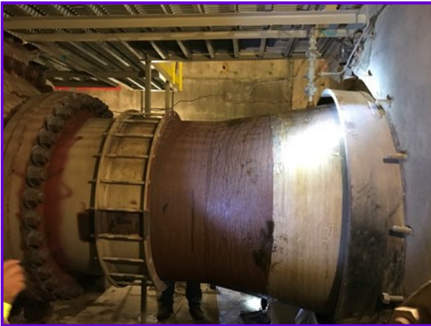
Left: Corroded 54-inch reducer in the Collis Avenue pressure regulating structure prior to replacement. Right: The new reducer installed in the Collis Avenue pressure regulating structure by the on-site contractor.
