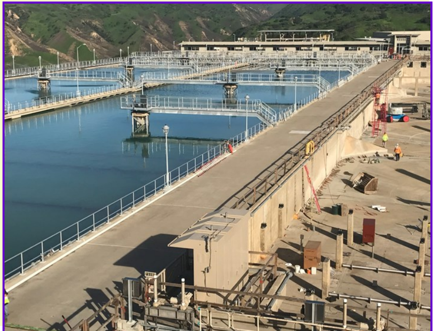
Diemer plant's recently rehabilitated basins in service with new equipment.
