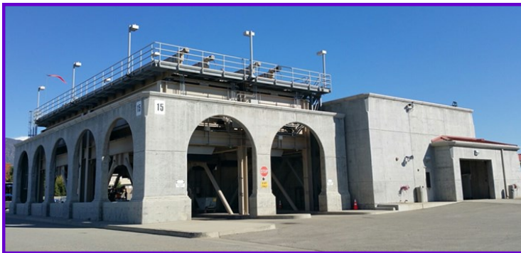
Solids Handling Building at Weymouth.
