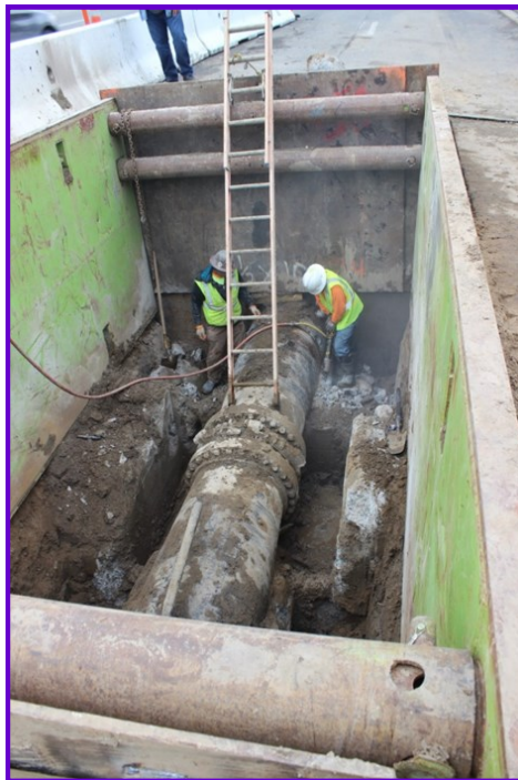
Orange County Feeder before (left) and after (right) the bulkhead installation to keep the majority of the feeder in service.
