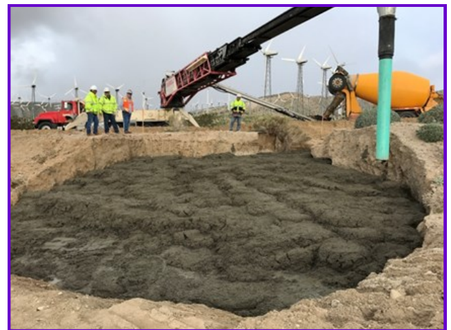
Slurry repairs
