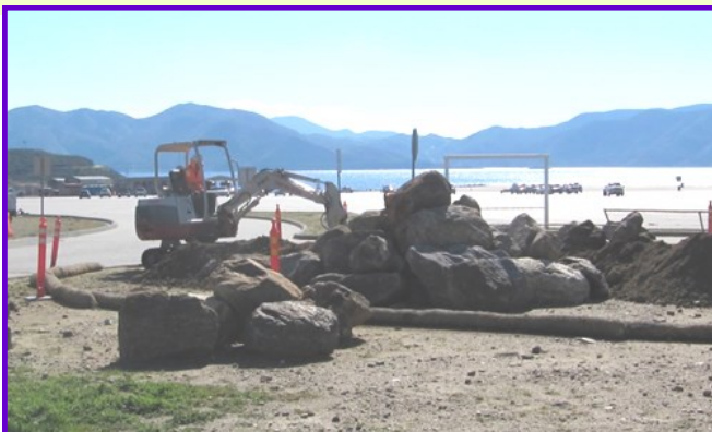
DVL East Dam Electrical Upgrades – Ductbank excavation at East Marina
