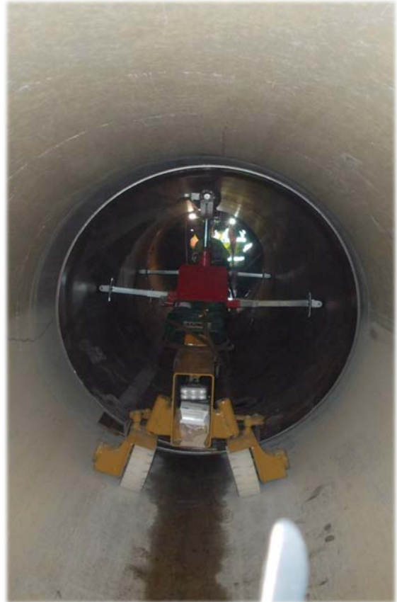
Second Lower Feeder Steel liner installation in 2015
