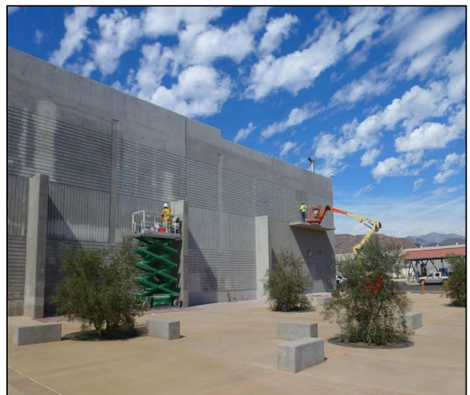
Weymouth Plant Ozone contactors
