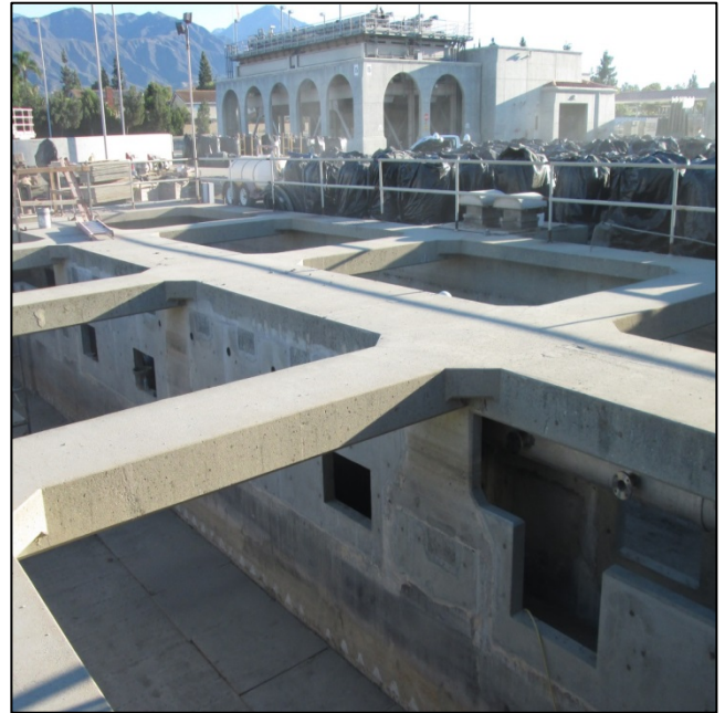
Weymouth Plant Concrete gullet wall repairs
