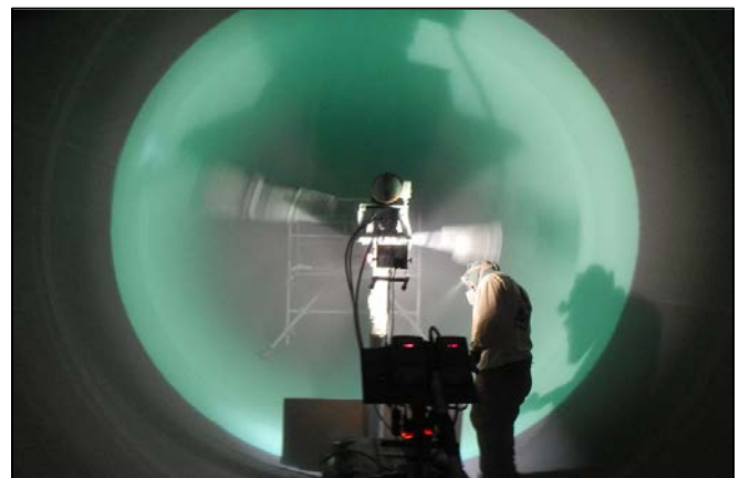
Etiwanda Pipeline Application of polyurethane coating
