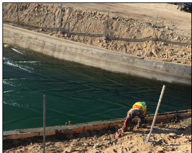
CRA Canal Concrete curbing at transition structure
