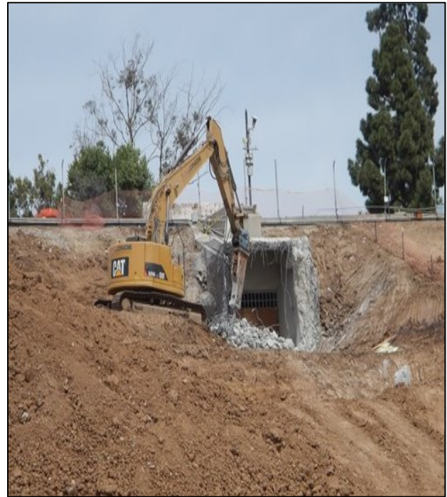
Palos Verdes Reservoir Demolition of reservoir overflow structure
