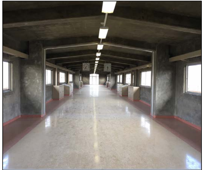
Diemer Plant East Filter Building
