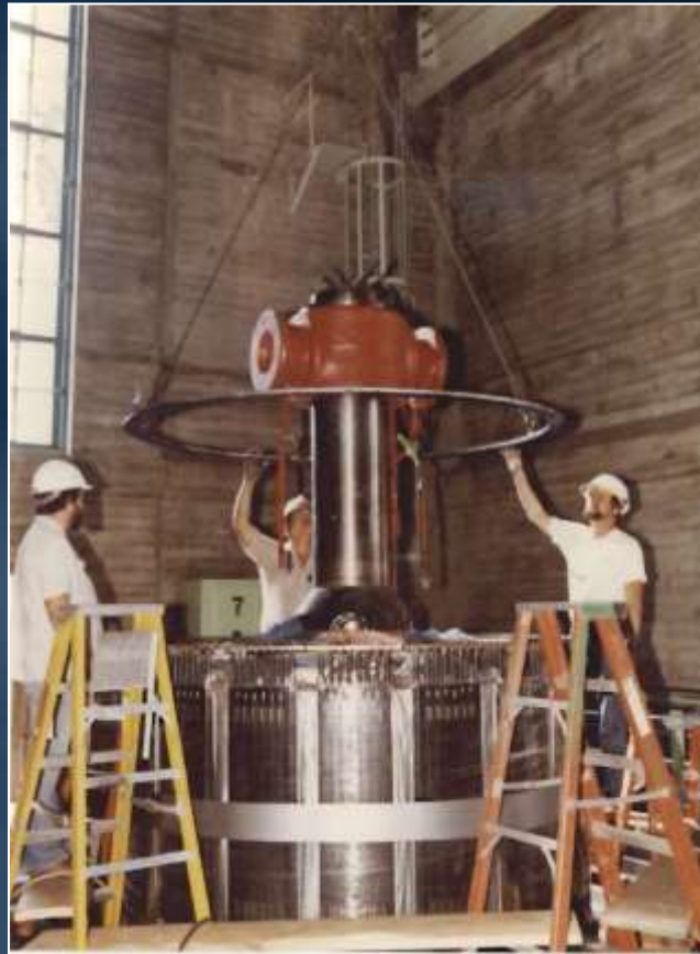
Re-assembling Rotor "Squirrel Cage"
