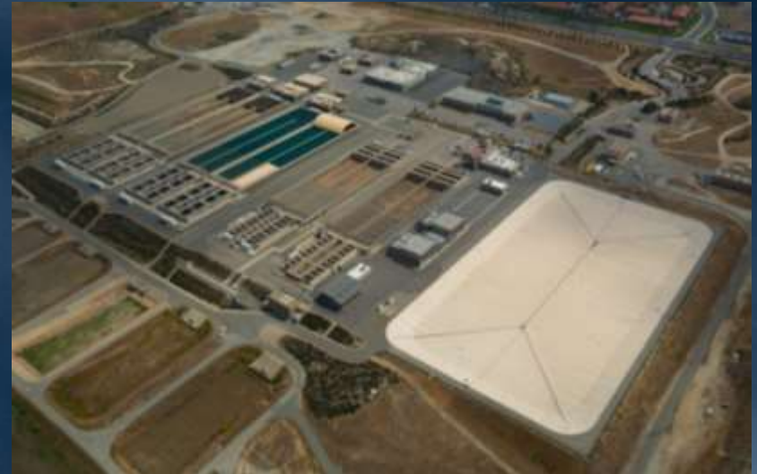
Finished Water Reservoir Covers
