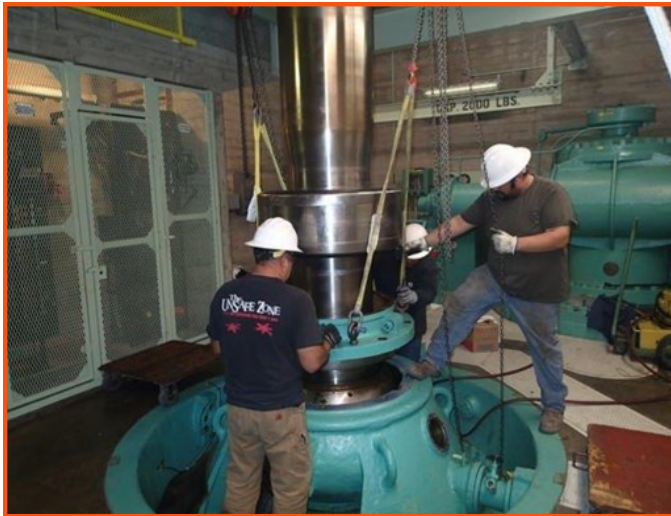
Disassembly of Pump Unit #3 at Intake Plant.
