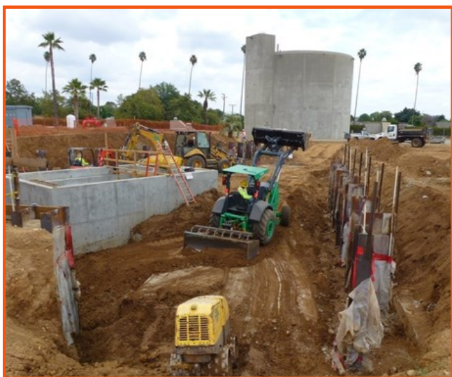
Weymouth ORP – Inlet bypass structure
