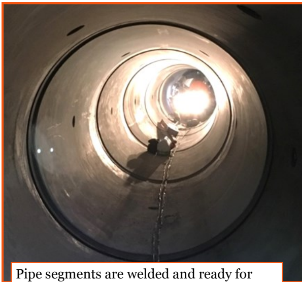
Welding of the pipe segments near Skirball Center Drive.
