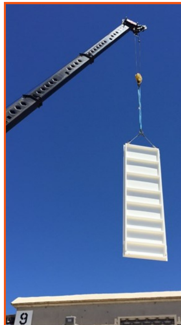
A gate being lowered using a crane (left) and (right) staff guiding the gate into the opening at the Jensen plant.
