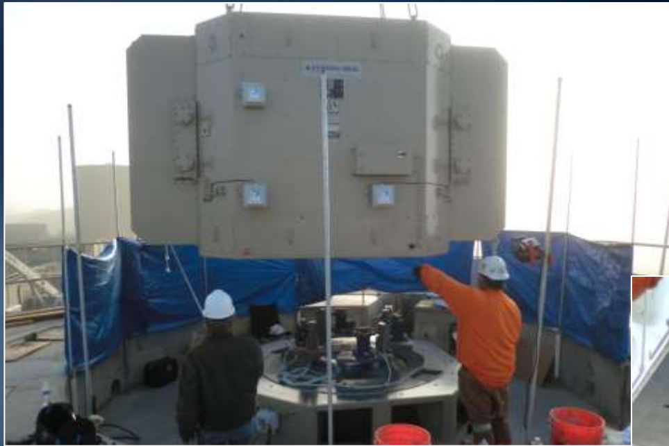
Positioning of generator main stator
