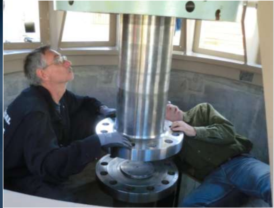
Positioning of rotor
