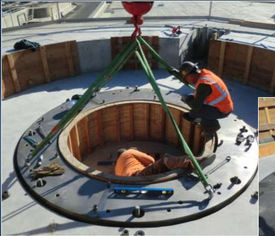
Positioning sole plate
