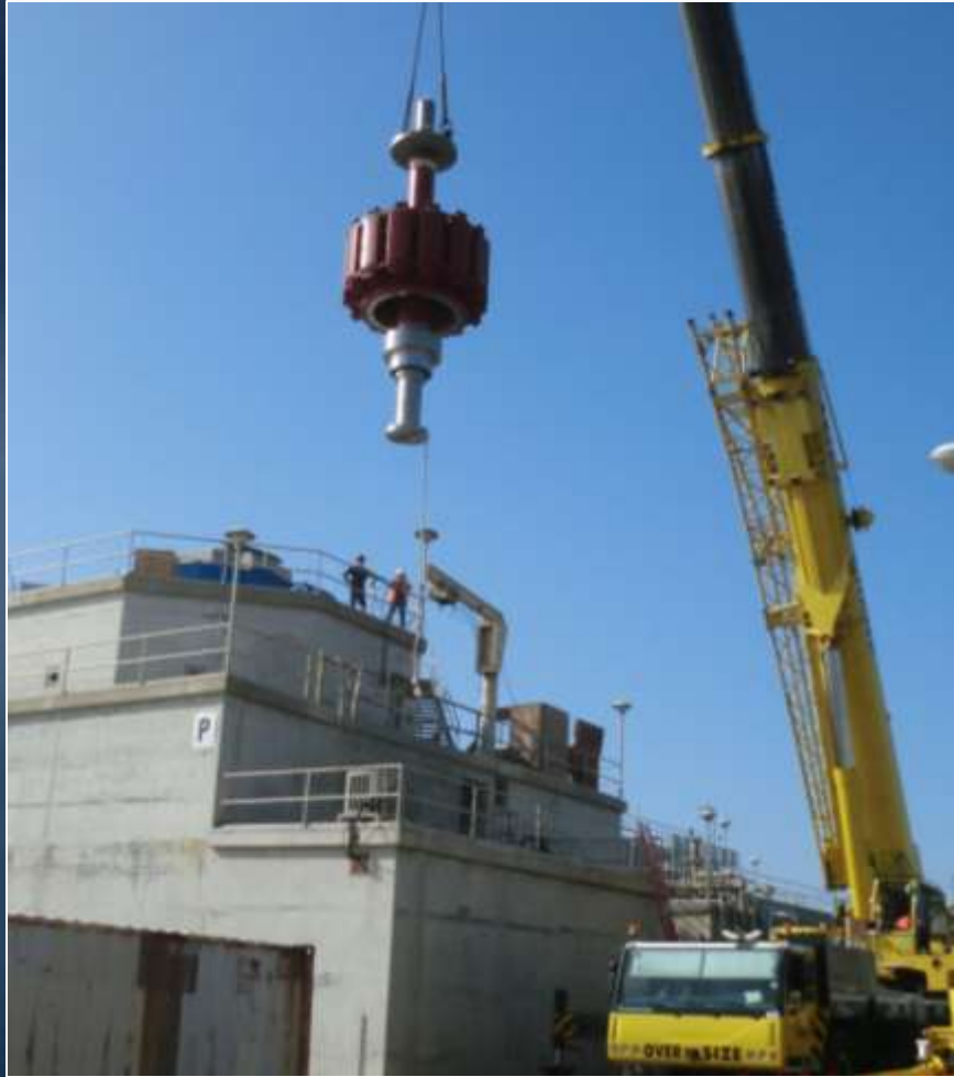
Crane placement of rotor
