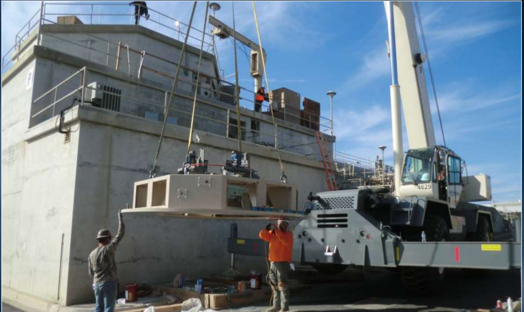
Crane – placement of generator lower bridge
