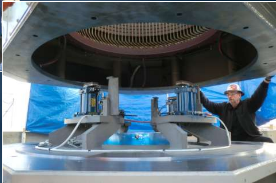
Positioning of generator main stator
