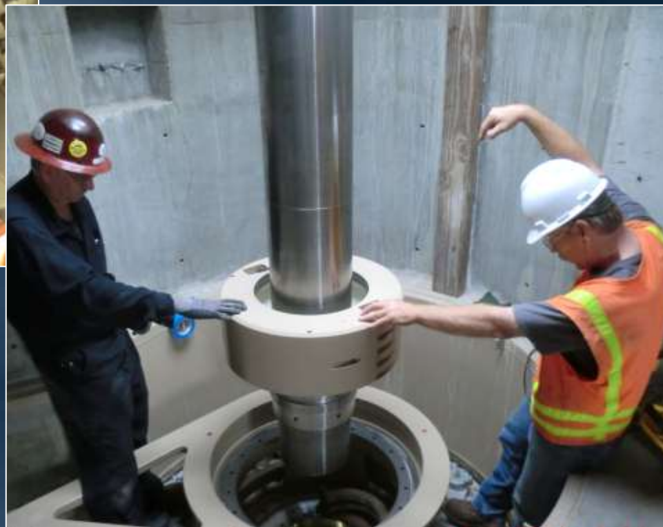
Installing turbine shaft
