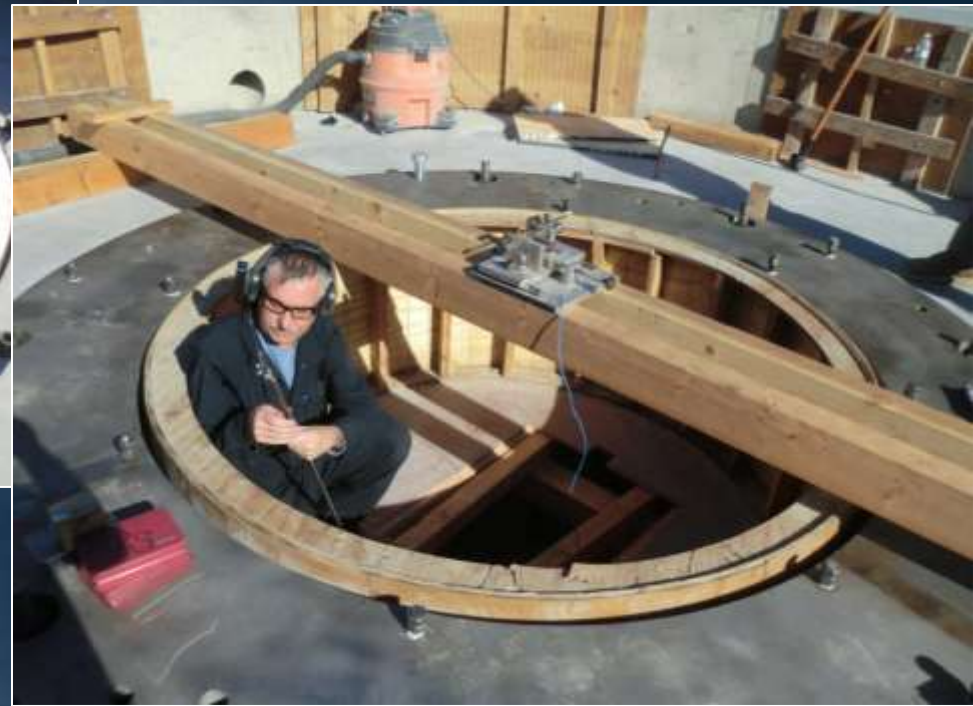
Checking sole plate alignment
