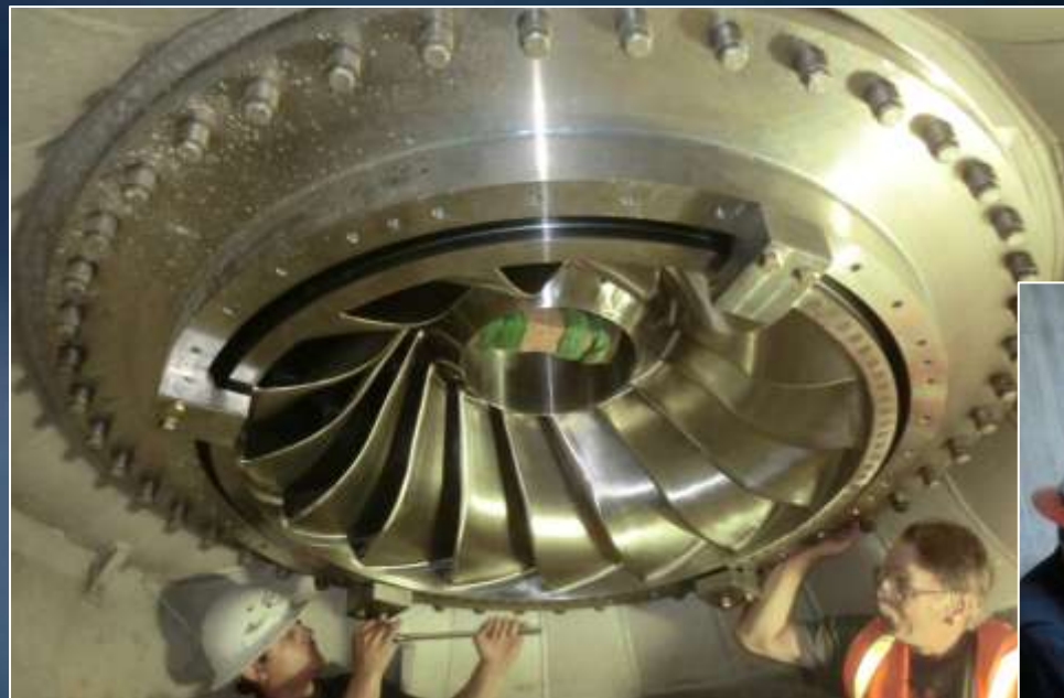
Installing new turbine runner
