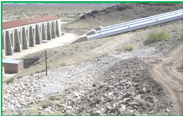
Re-grading of access roads and rock placement
