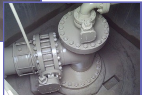
Before (above) and after (below) coating work at San Diego Pipeline 5
