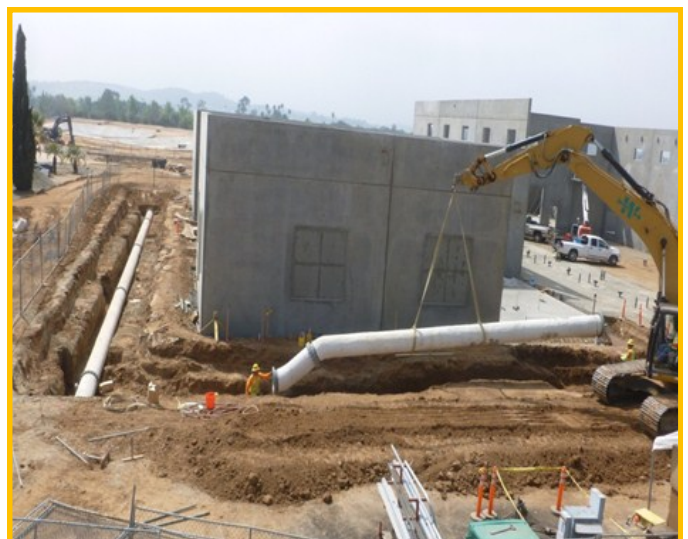
Weymouth ORP—Installation of Cooling Water Pipe Story on page 5.
