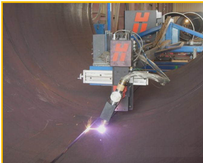
PCCP Repair—Trimming Seam of Collapsible Steel Liner Story on page 6.
