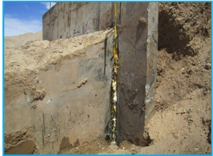
Repaired leak site after sealant injected into joint
