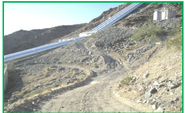
Added drainage channels
