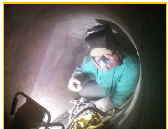
Welding the 12-inch diameter steel plate
