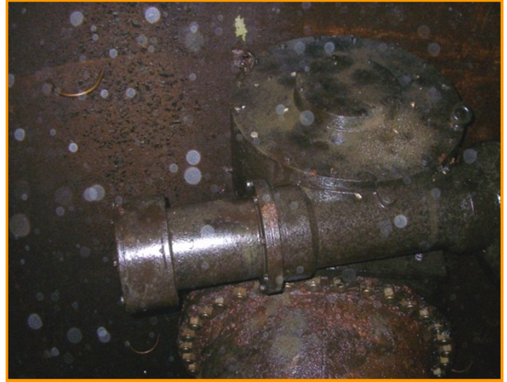
After cleaning: Chlorine shock treatment and pressure washing
