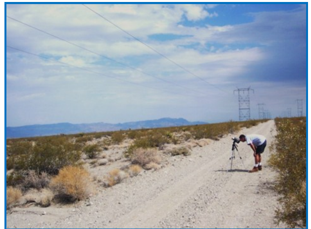
Performing thermographic surveys on the East and West 230kV Mead-Camino transmission lines
