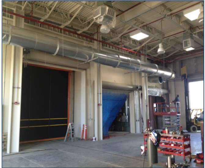
La Verne Coating Shop New ventilation ductwork
