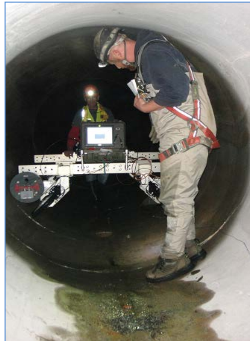
Second Lower Feeder Electromagnetic inspection
