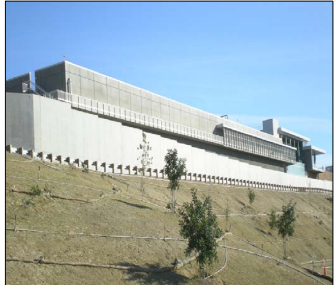
Diemer Plant Ozone Generation Building and Contractors
