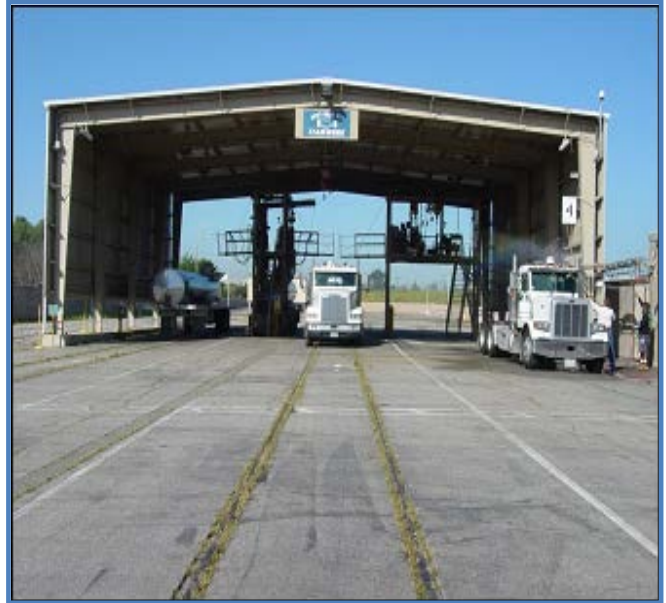
Existing Chemical Unloading Facility
