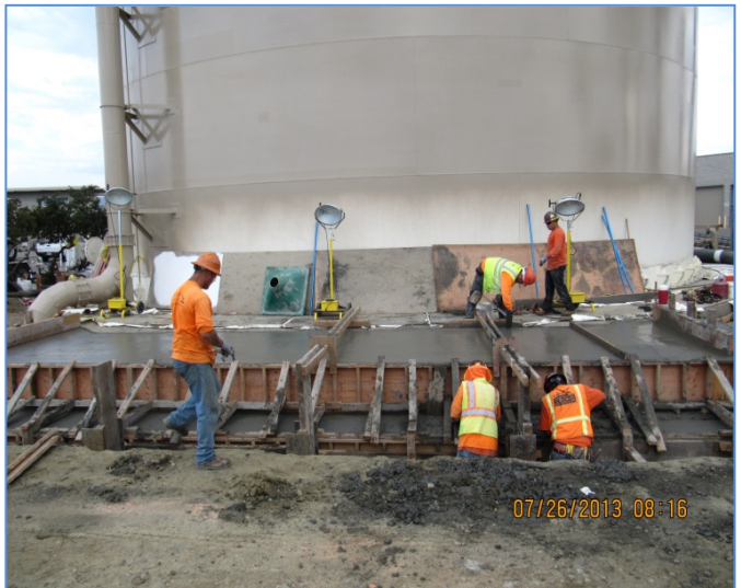
Diemer Plant Concrete placement on south shearwall
