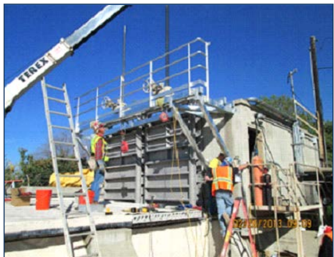
Upper Feeder Gate installation at Puddingstone Spillway
