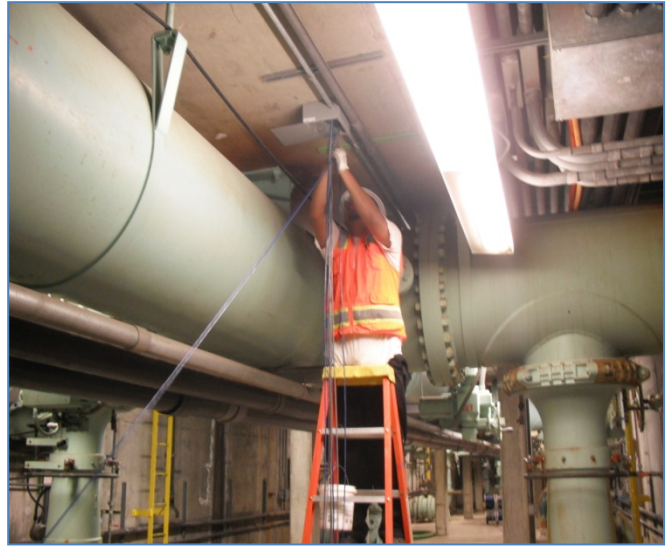
Weymouth Plant Speaker cable/wire installation inside the filter pipe gallery
