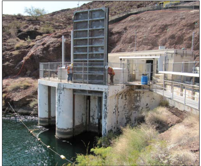
Copper Basin Reservoir Outlet Structure Installation of refurbished slide gate
