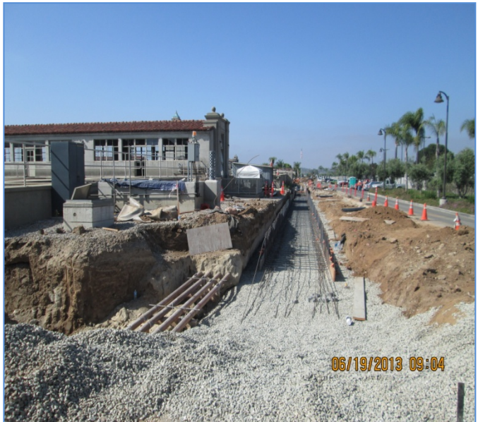
Weymouth Plant Reinforcing steel placement for the chemical trench
