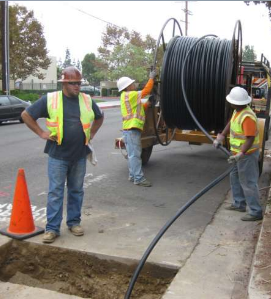
Installing Cable to Anodes
