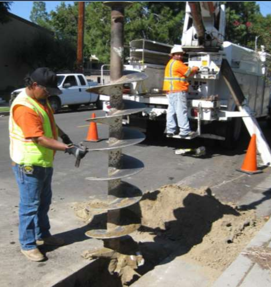
Drilling Borings
