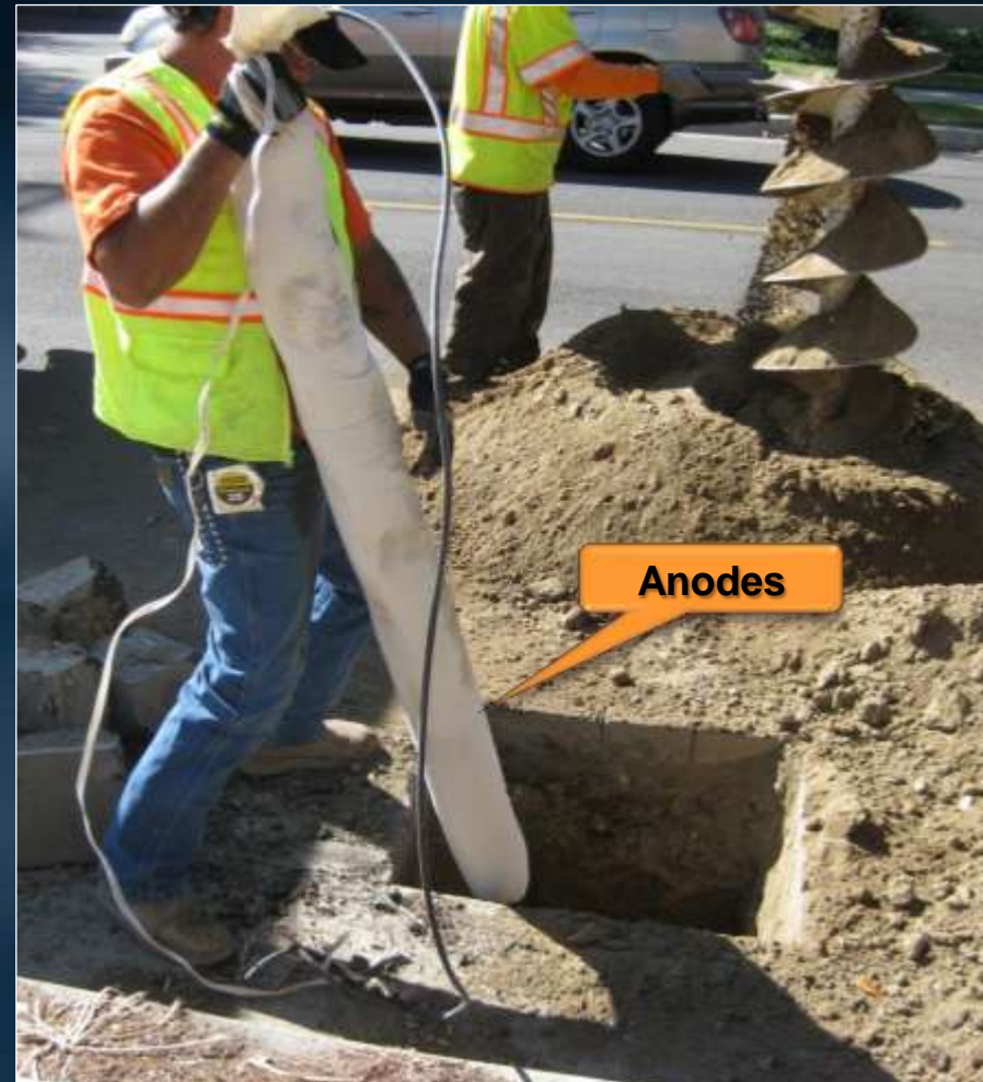
Installing Anodes
