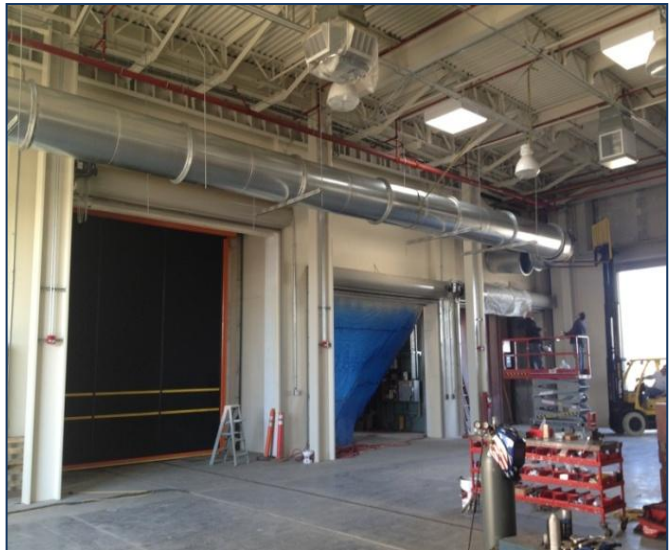
La Verne Coating Shop New ventilation ductwork
