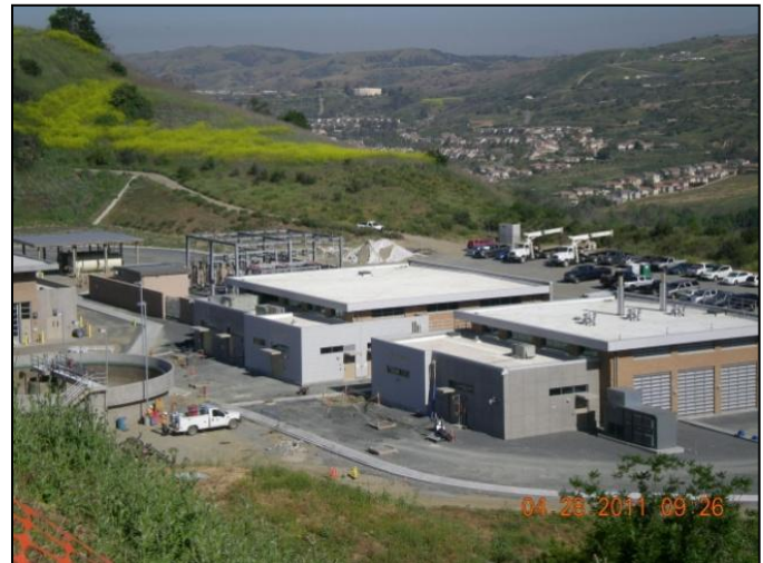
Diemer Plant New switchgear and standby generator buildings
