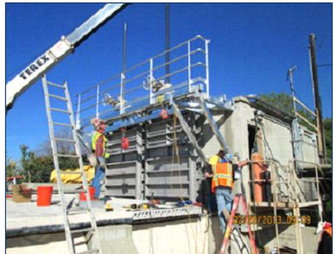
Upper Feeder Gate installation at Puddingstone Spillway
