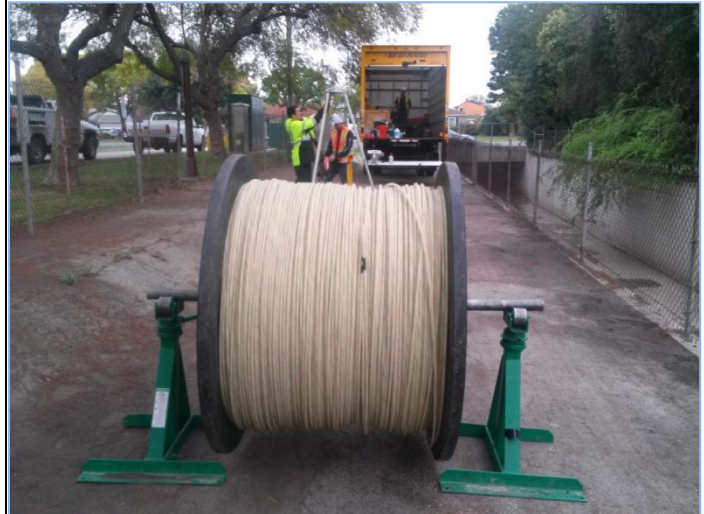
Second Lower Feeder Installation of Acoustic Fiber Optic monitoring system
