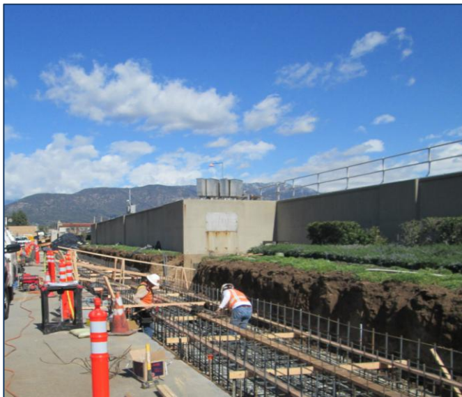
Weymouth Plant Reinforcing steel placement for the chemical trench
