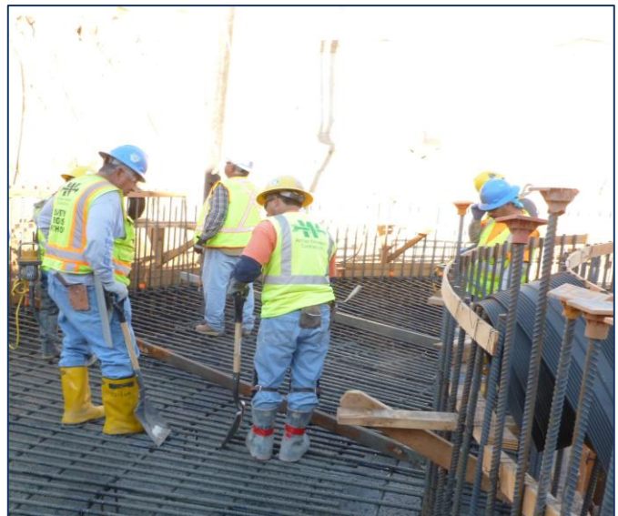
Weymouth Plant Placement of concrete for ozone contactor outlet structure
