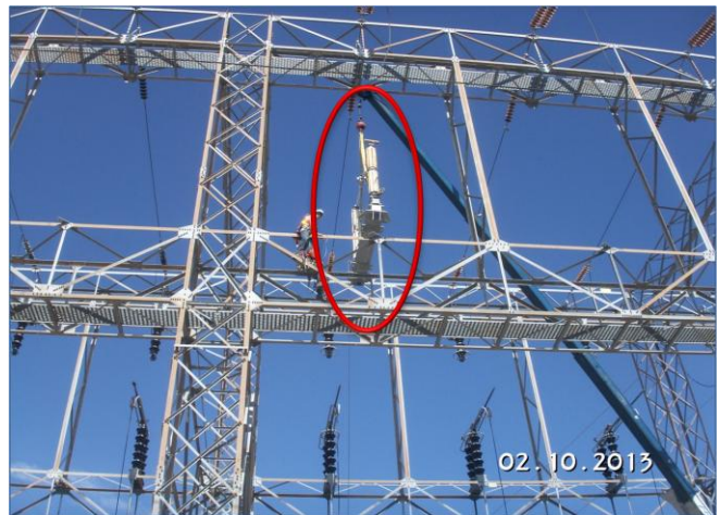
CRA Pumping Plants High voltage disconnect switch replacement
