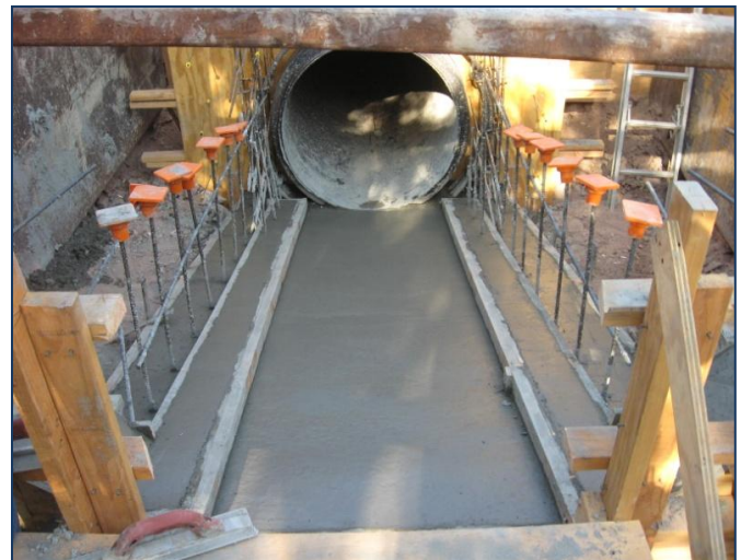
Concrete placement of storm drain inlet
