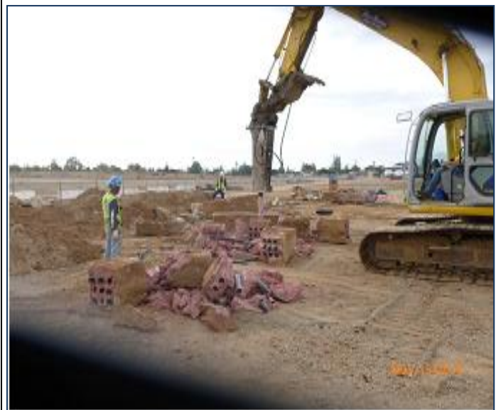
Weymouth Plant Electric duct bank removal
