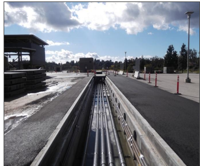
Jensen Plant New chemical trench and chemical feed piping
