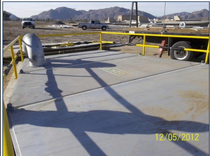
Colorado River Aqueduct Transition structure covers
