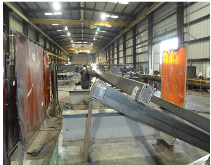
Fabrication of new components in the contractor’s shop
