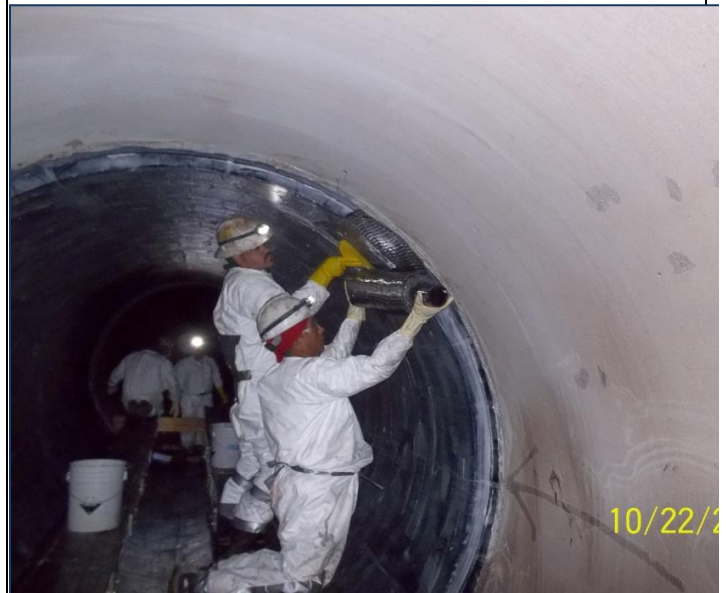
Application of carbon fiber lining on San Diego Pipeline No. 5
