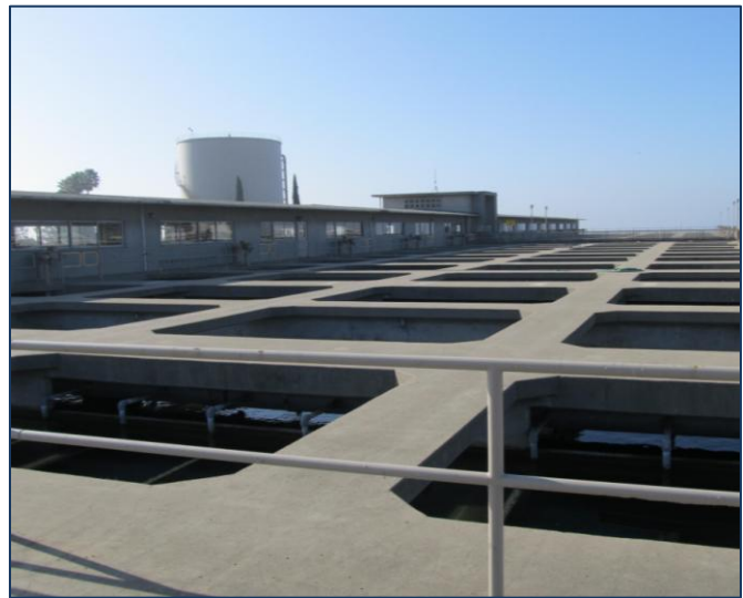
Diemer Plant Filters in east module
