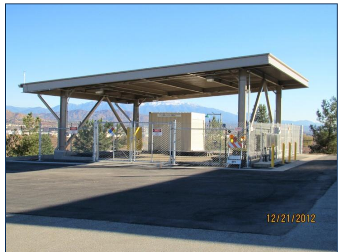
Mills Plant Hazardous Waste Staging and Containment Facility
