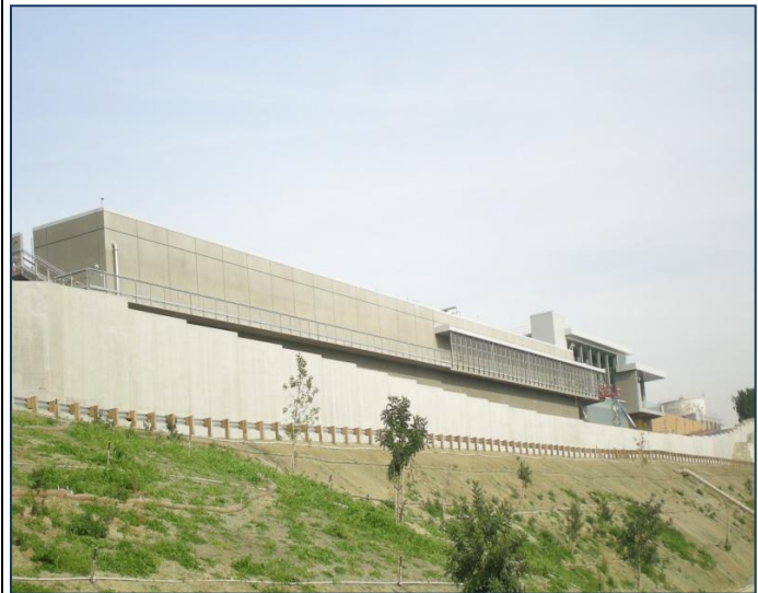
Diemer Plant Ozone Generation Building and Contactors
