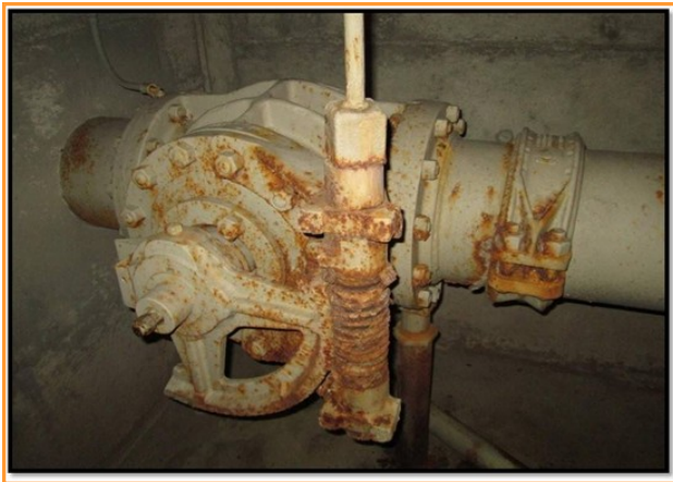
Orange County Feeder turn-out valve (OC-7) before and after coating
