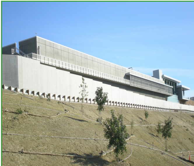
Diemer Ozone Generation Building and Contactors
