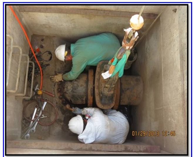
Staff removing San Diego Pipeline No. 1 turn-out valve
