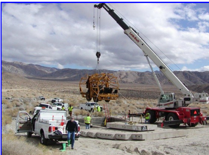
Staff setting up the tunnel cleaning equipment for the CRA shutdown
