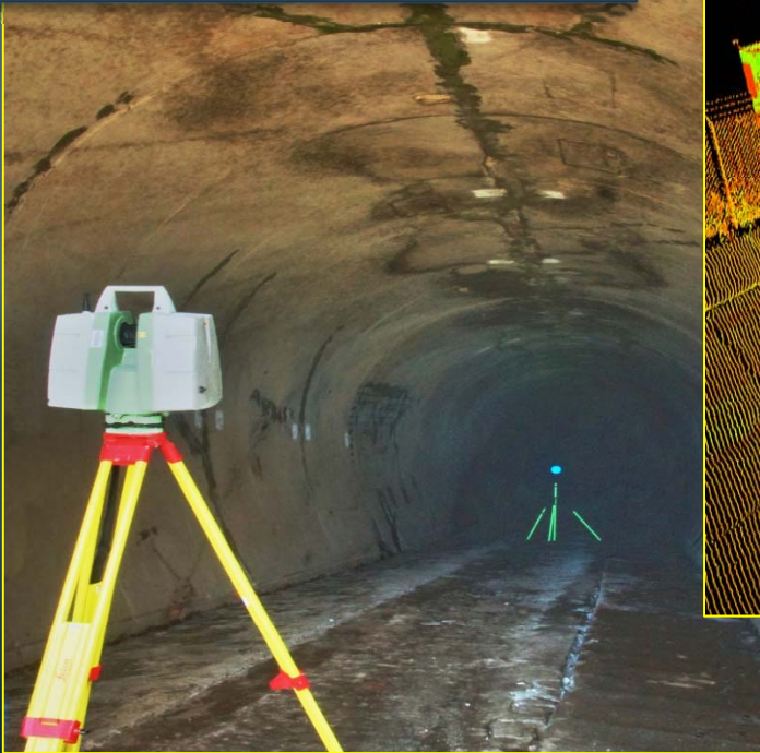
Survey of San Fernando Tunnel
