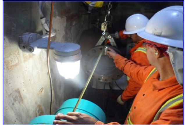
Working on new bypass for Glendale
