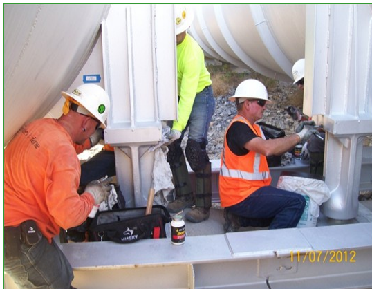
Replacement of support bolts on CRA pump plant delivery lines
