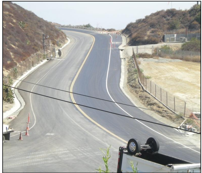
Diemer Plant Main entrance road improvements
