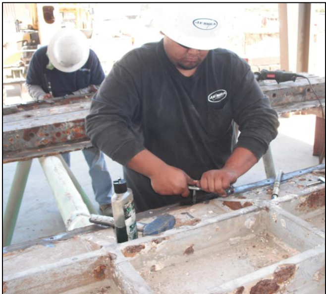
Refurbishment of Eagle Rock Gates
