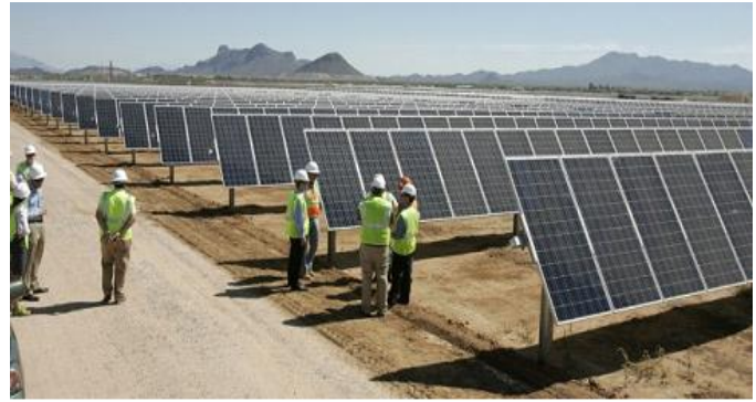
SunEdison Solar Farm in Tucson, AZ
