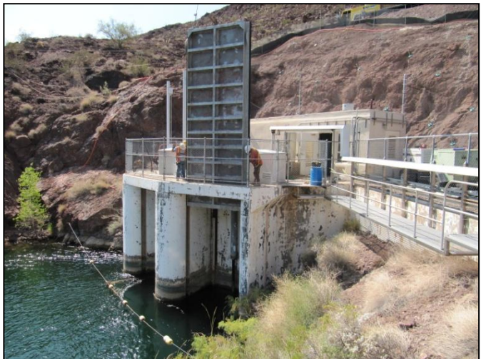
Copper Basin Reservoir Outlet Structure Installation of refurbished slide gate
