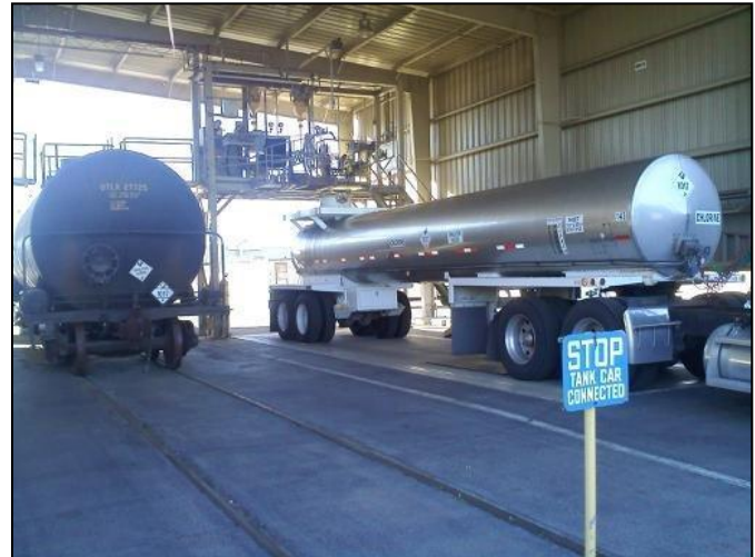
Existing Chemical Unloading Facility
