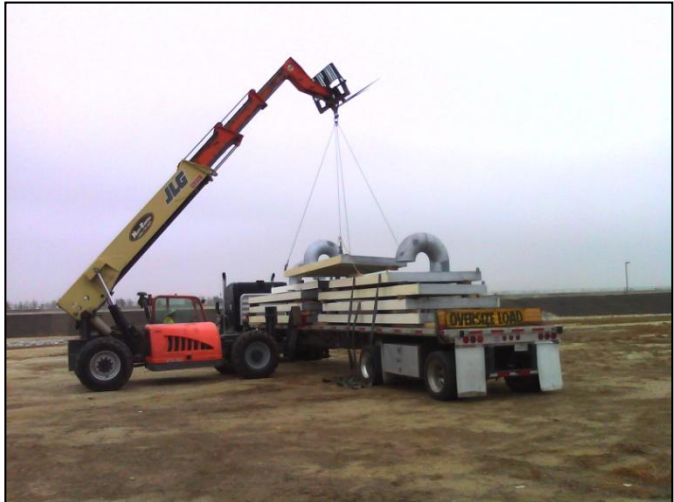
Colorado River Aqueduct - Unloading of transition structure covers
