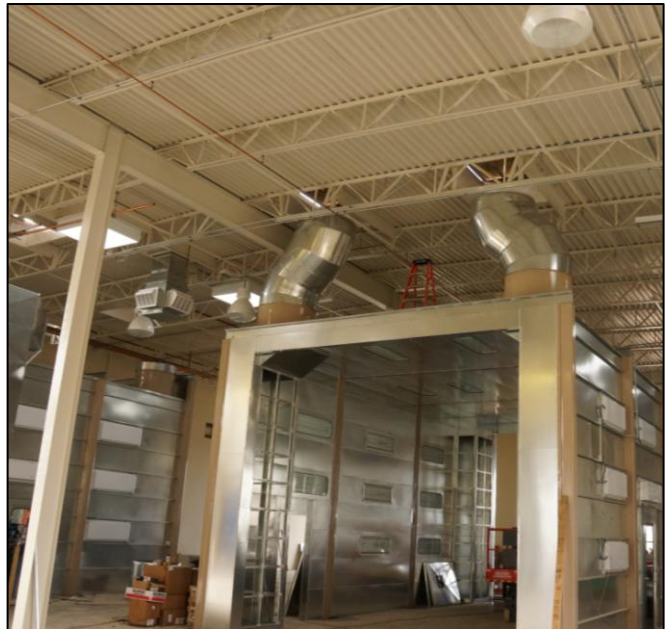
La Verne Coating Shop New blast booth
