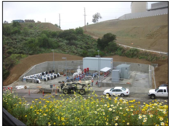
Diemer Plant Fire and potable water pump station
