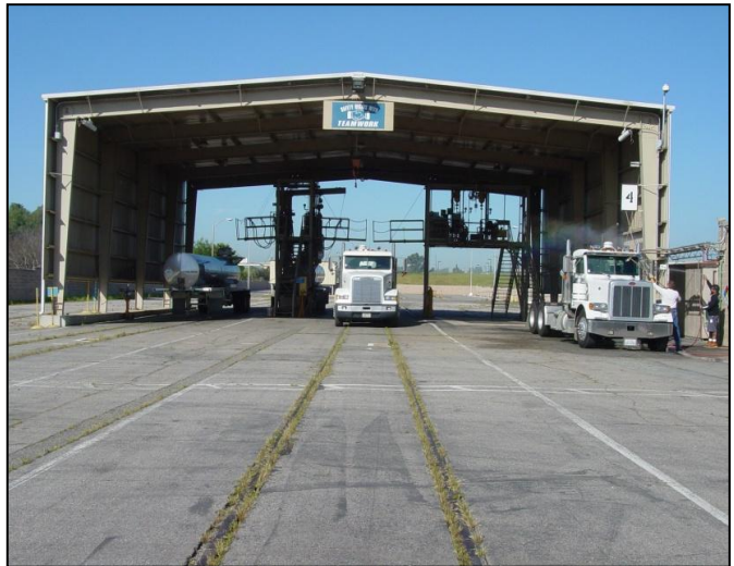
Existing Chemical Unloading Facility
