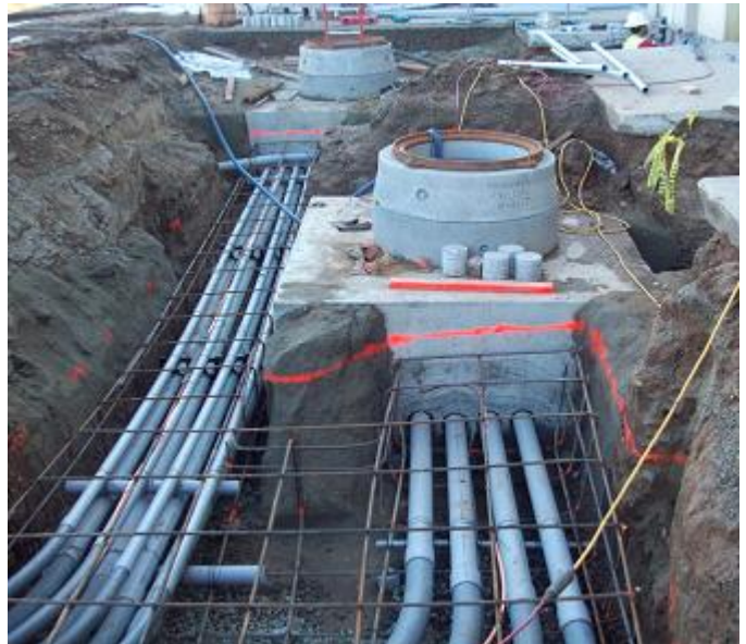
LaVerne Coating Shop New electrical duct bank and manhole
