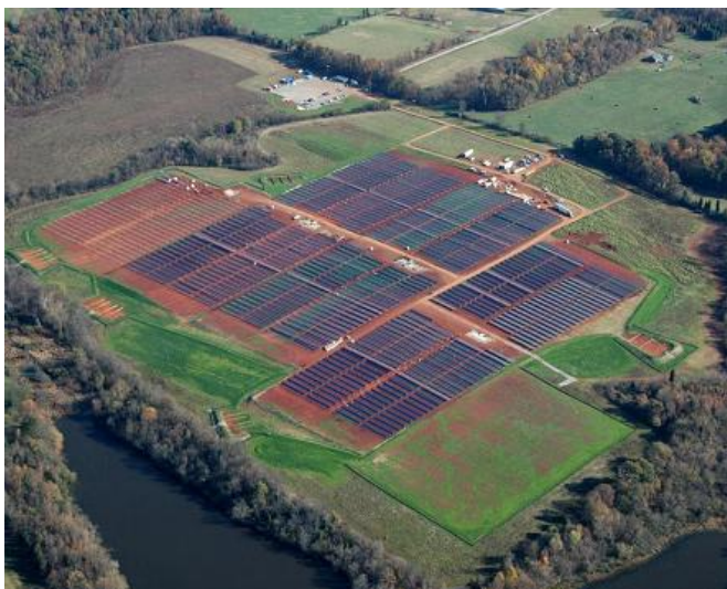
SunEdison solar farm in North Carolina
