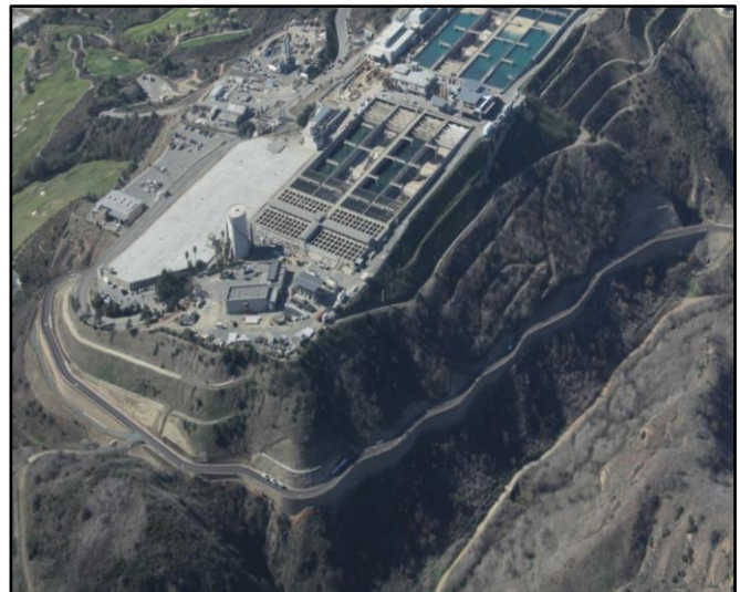
Diemer North Access Road
