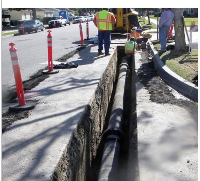
Installed piping in trench in City of Downey
