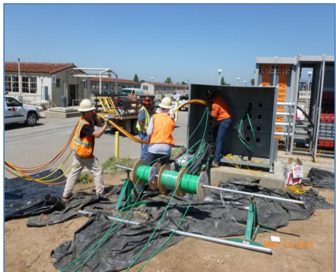
Weymouth Plant Electrical cable installation
