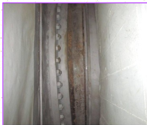
The 72-inch expansion joint at Gene unit No. 4 before corrosion repairs (top) and after refurbishment (below)
