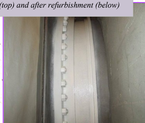
The 72-inch expansion joint at Gene unit No. 4 before corrosion repairs (top) and after refurbishment (below)
