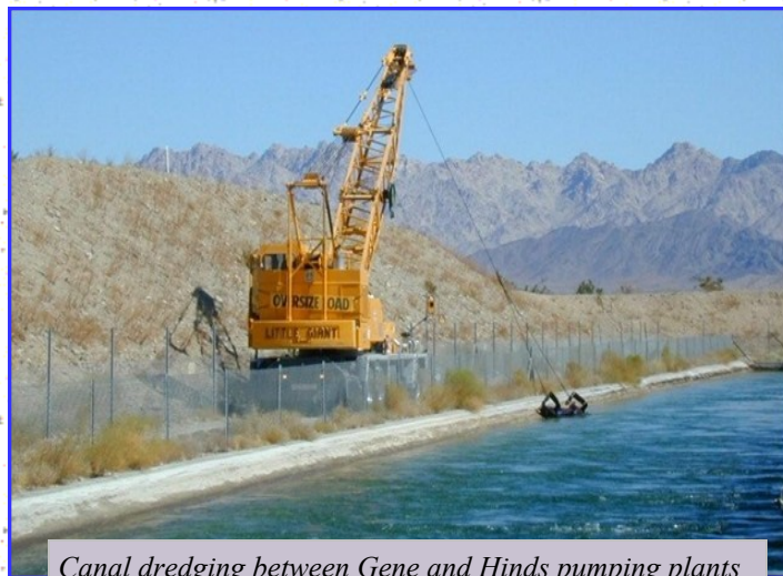
Canal dredging between Gene and Hinds pumping plants
