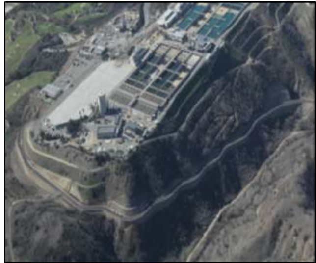
Diemer North Access Road
