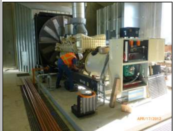
Weymouth Power System Upgrade Standby Generator Installation
