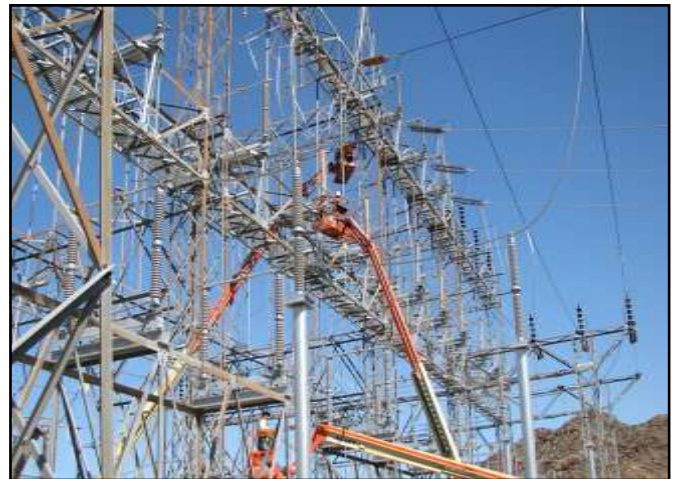
CRA High Voltage Disconnect Switches Replacement
