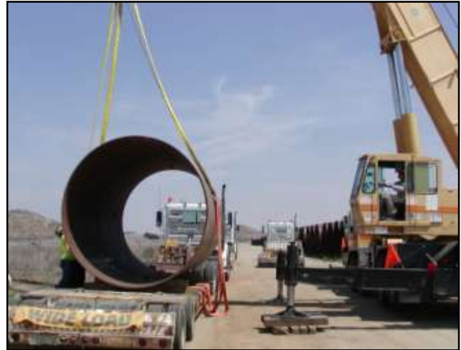
Metropolitan crews unloading tunnel casing for storage at Lake Mathews
