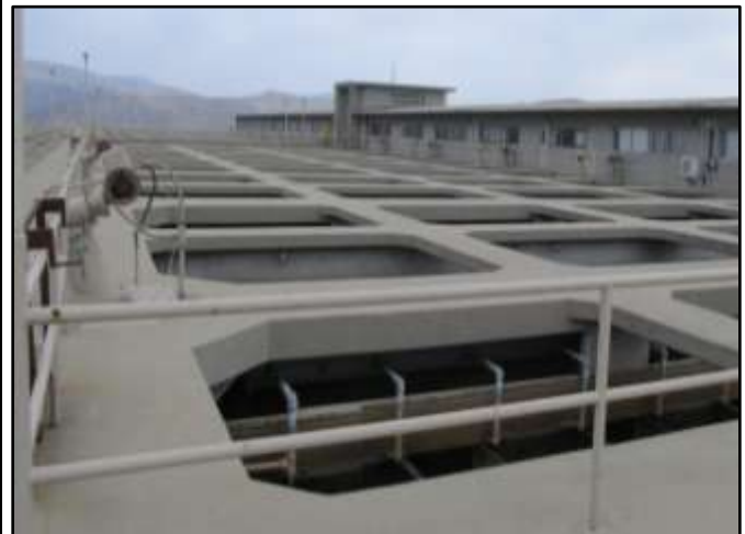
Diemer Plant West-Side Filter Bays
