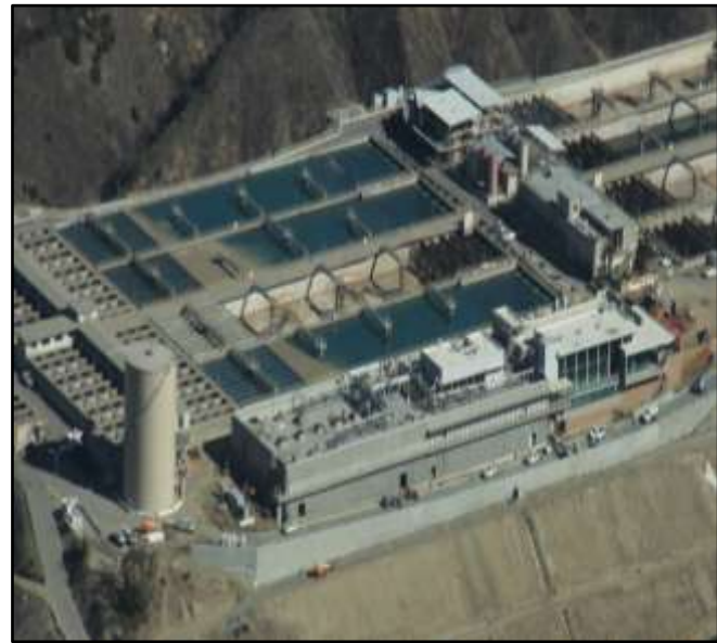
Diemer Plant New Ozone Generation Building and Contactors
