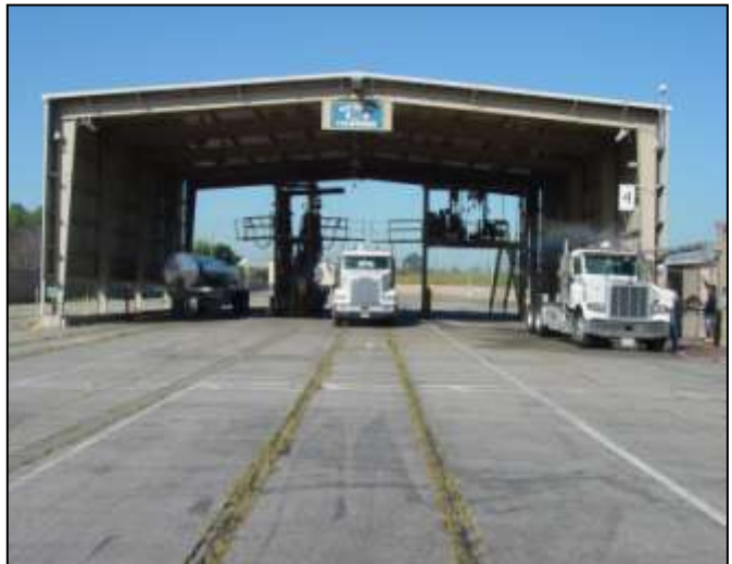
Existing Chemical Unloading Facility
