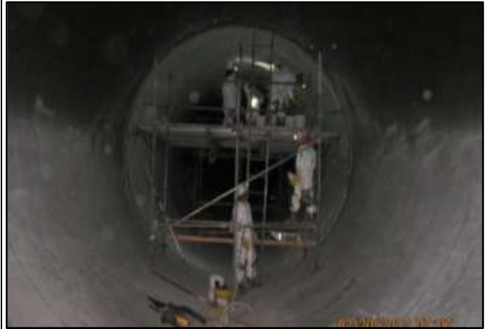
PCCP Rehabilitation Carbon Fiber Joint Repairs
