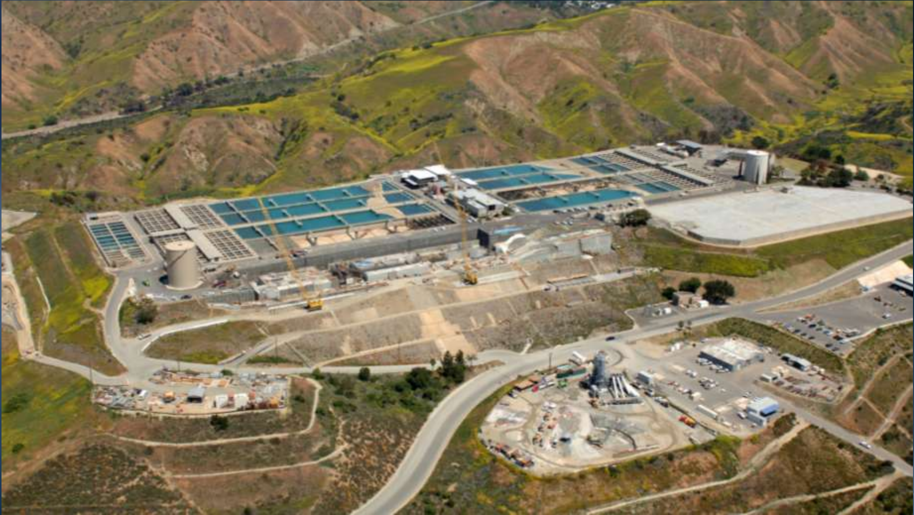
Diemer WTP - April 2009
