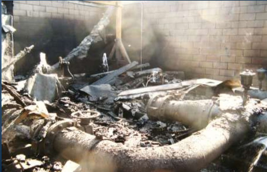
OC-71 Service Connection Structure - 2007
