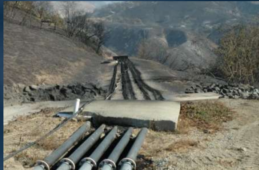
Fiber Optic Cable at Diemer - 2008
