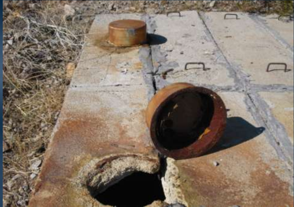
Existing septic tanks at Hinds P.P.
